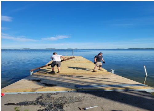
Installing new JMP pier
