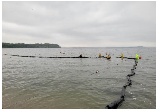
Installing Warner Park beach curtain
