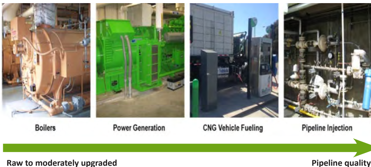
FIGURE 21: BIOGAS PURIFICATION LEVELS AND ASSOCIATED USES
