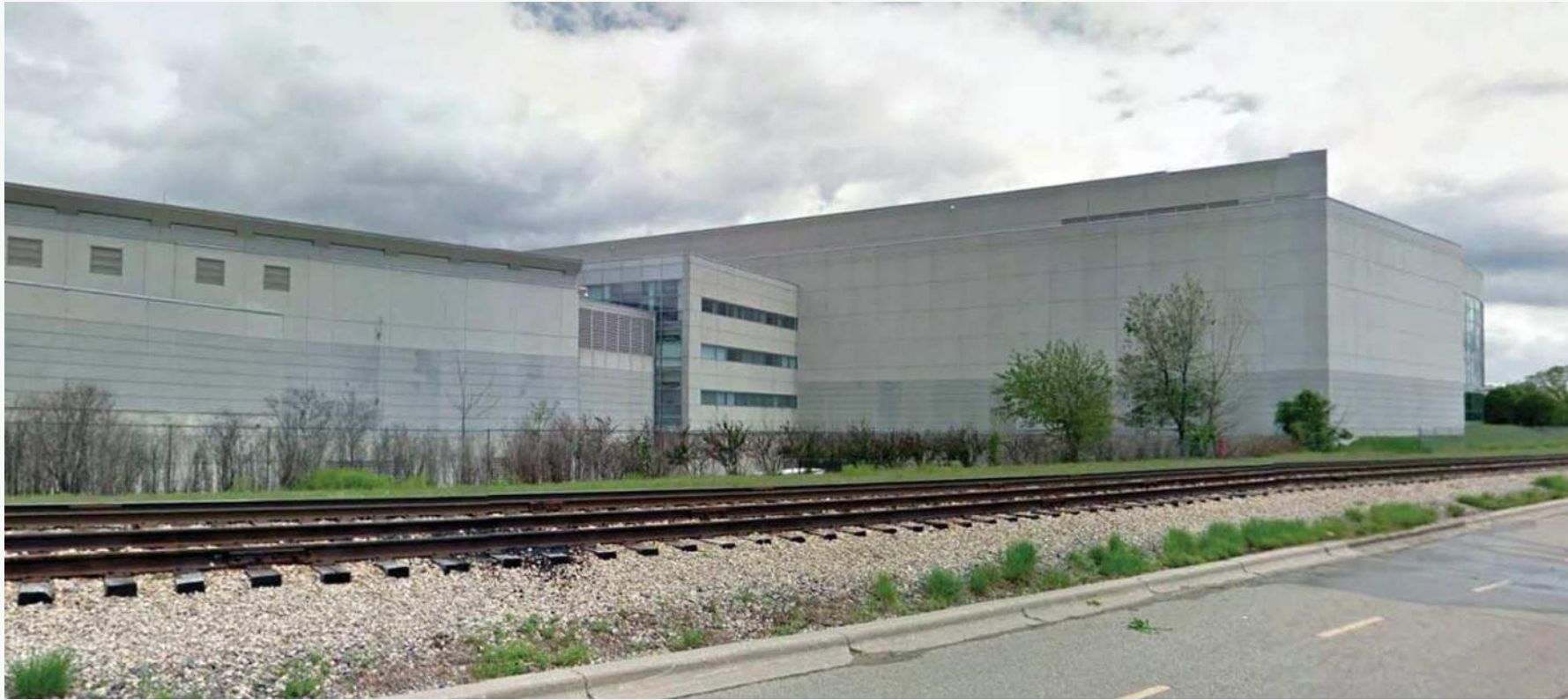
Existing southwest corner/facade view from commuter bike path
