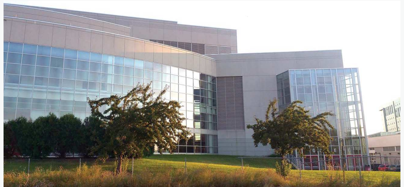
Existing southeast corner/facade view from commuter bike path
