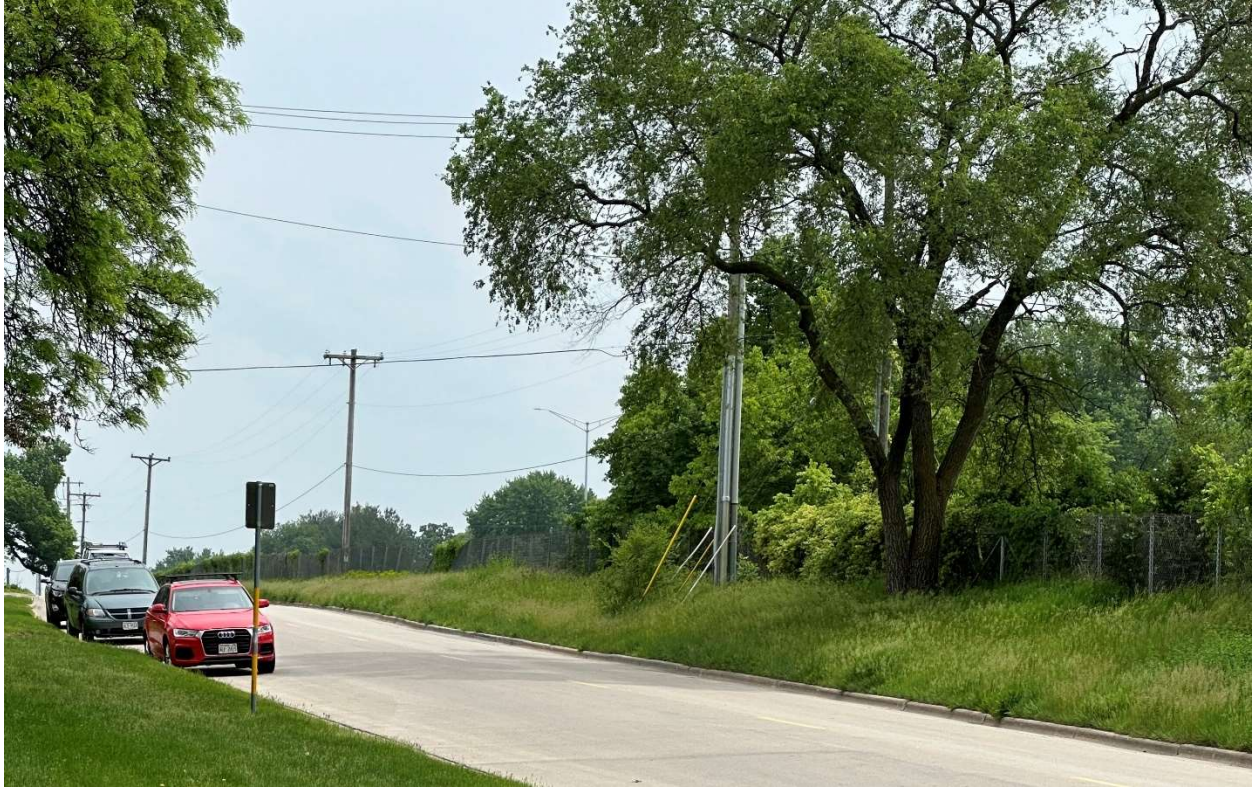
(S Stoughton Rd leading to the proposed site)
