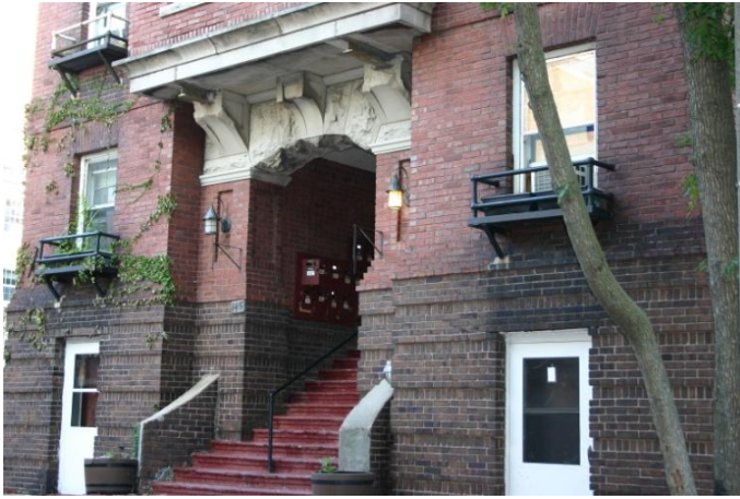
Front entrance of 145 Iota Court – proposed for demolition
