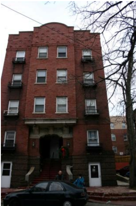
145 Iota Court – proposed for demolition
