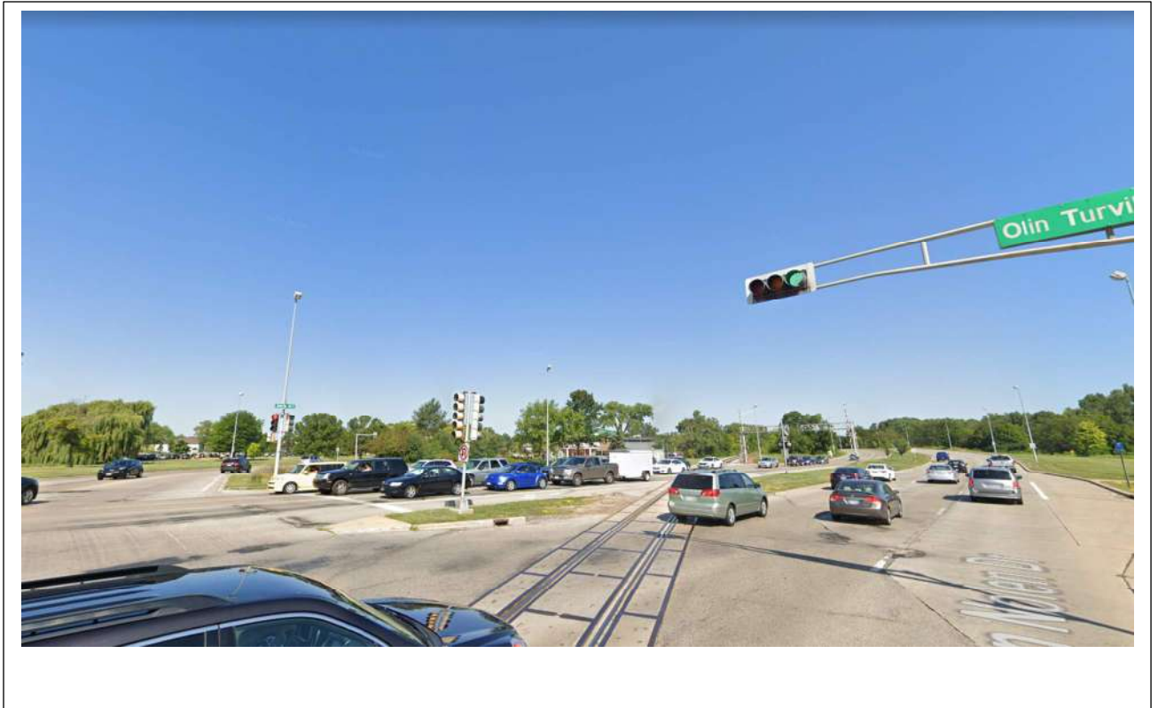
Olin – Turnville CT – Facing West
