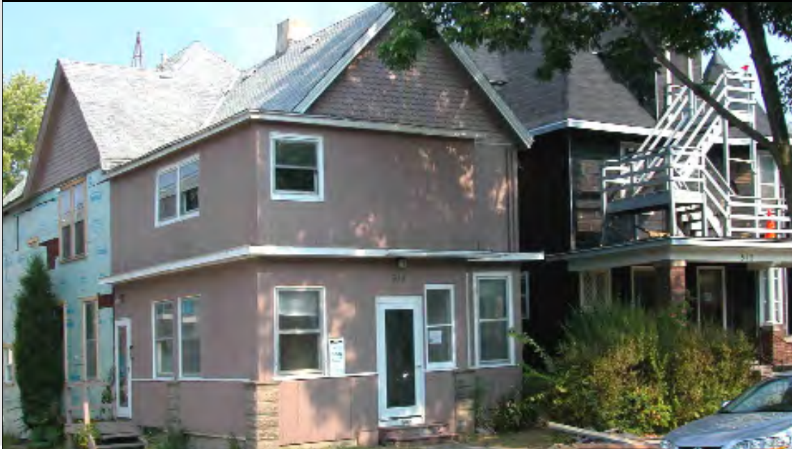
A MODERN ADDITION THAT ALTERS THE ORIGINAL CHARACTER OF THE BUILDING AND INCLUDES AN INTRUSIVE SECOND EXIT STAIR
