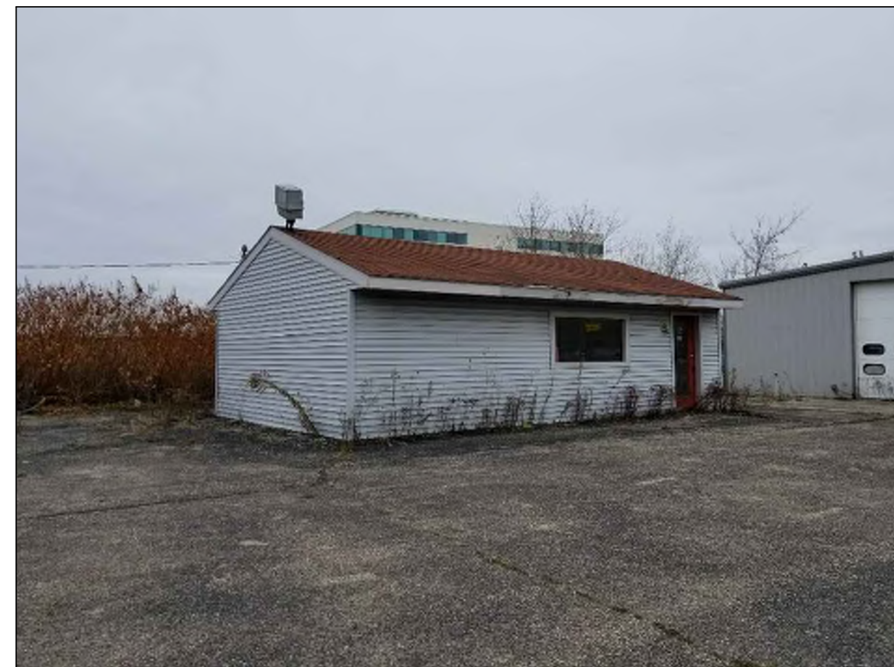
CENTER OF SOUTH SIDE LOOKING NORTHEAST
