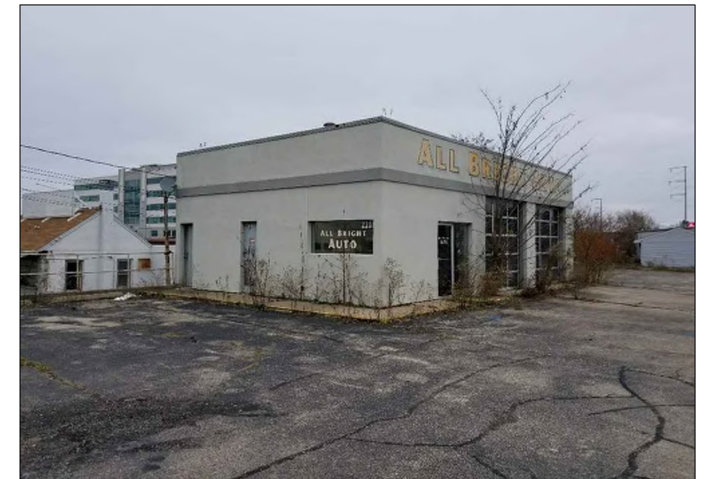
SOUTHWEST CORNER LOOKING NORTHEAST
