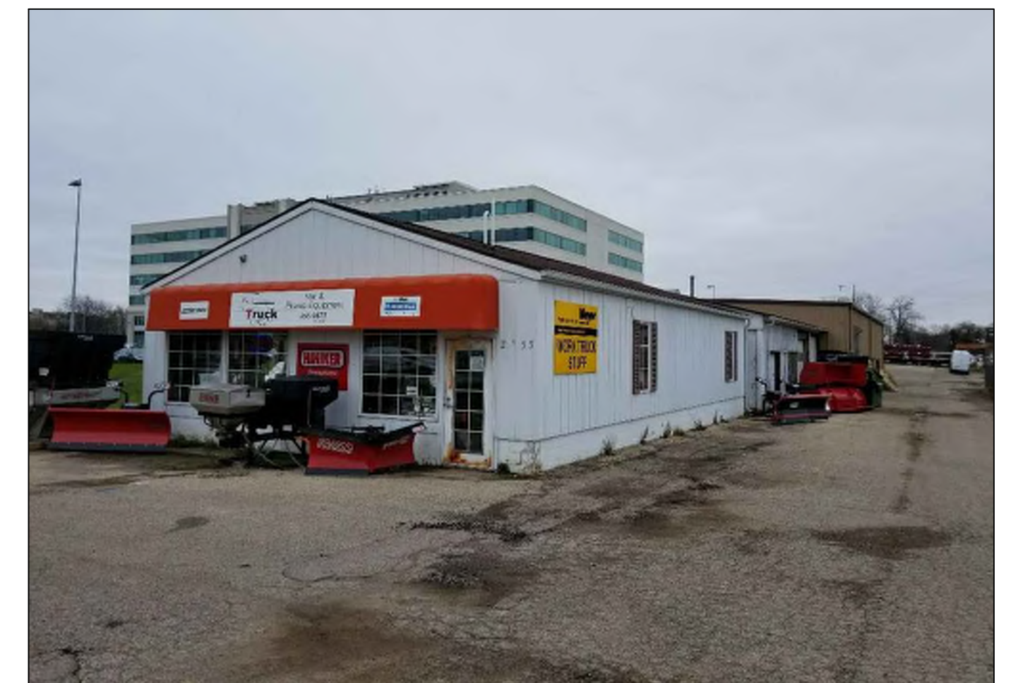
NEAR NORTHWEST CORNER LOOKING NORTHEAST
