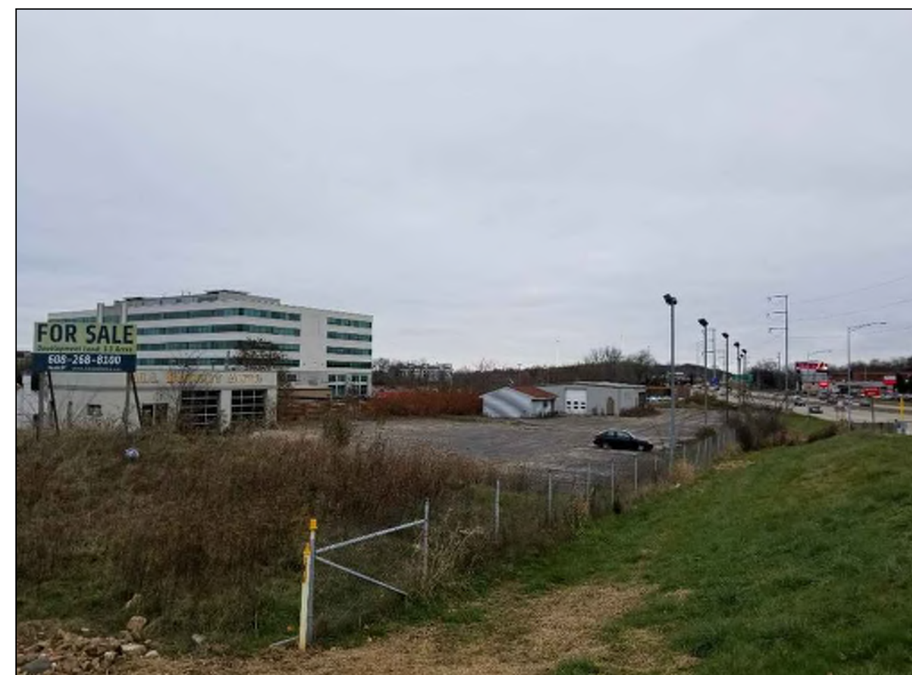
SOUTHWEST CORNER LOOKING NORTHEAST
