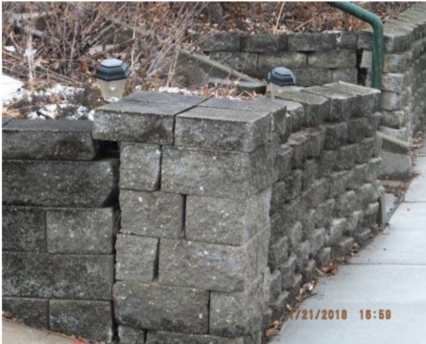
Sidewalk built around wall
