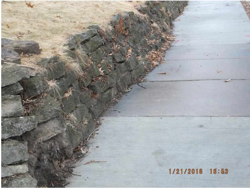
Sidewalk built around wall
