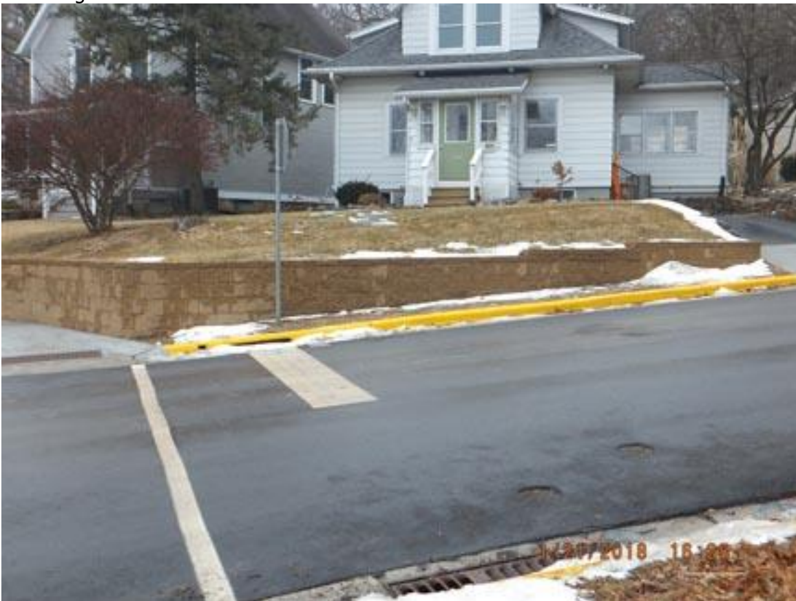
Retaining wall at 520 Sheldon constructed in 2017:
