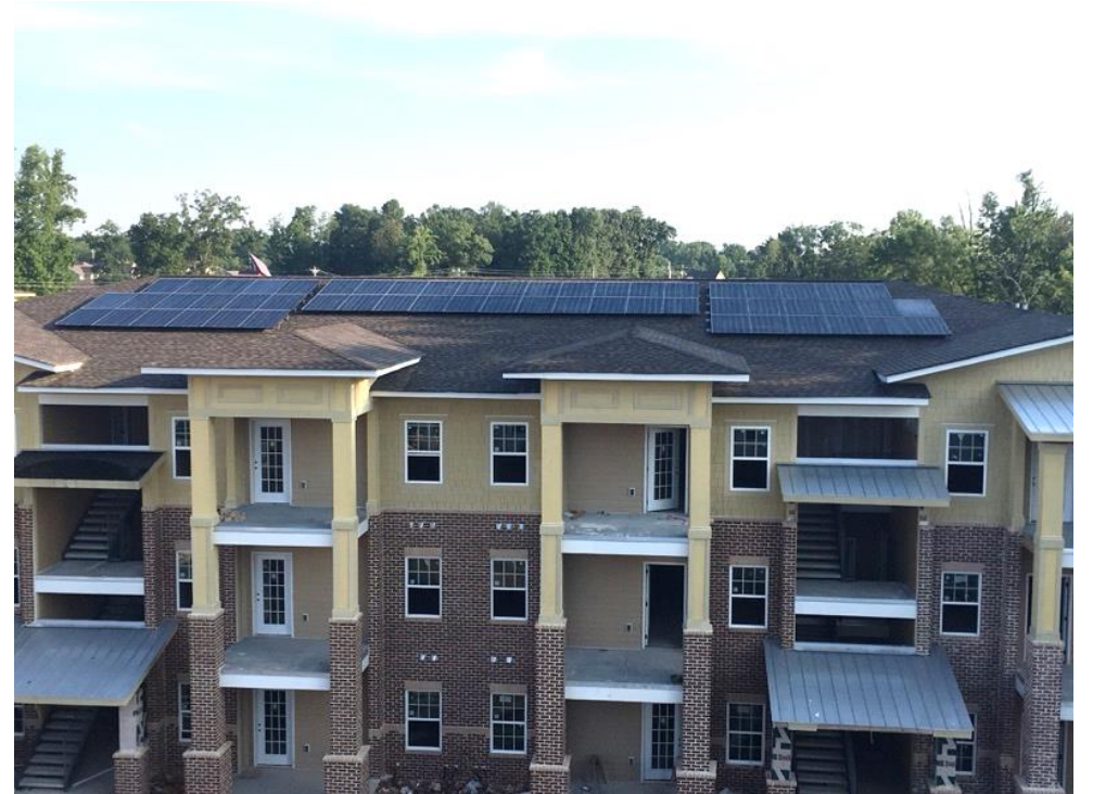
30kw solar PV system on multifamily housing building (Lightwave Solar)
