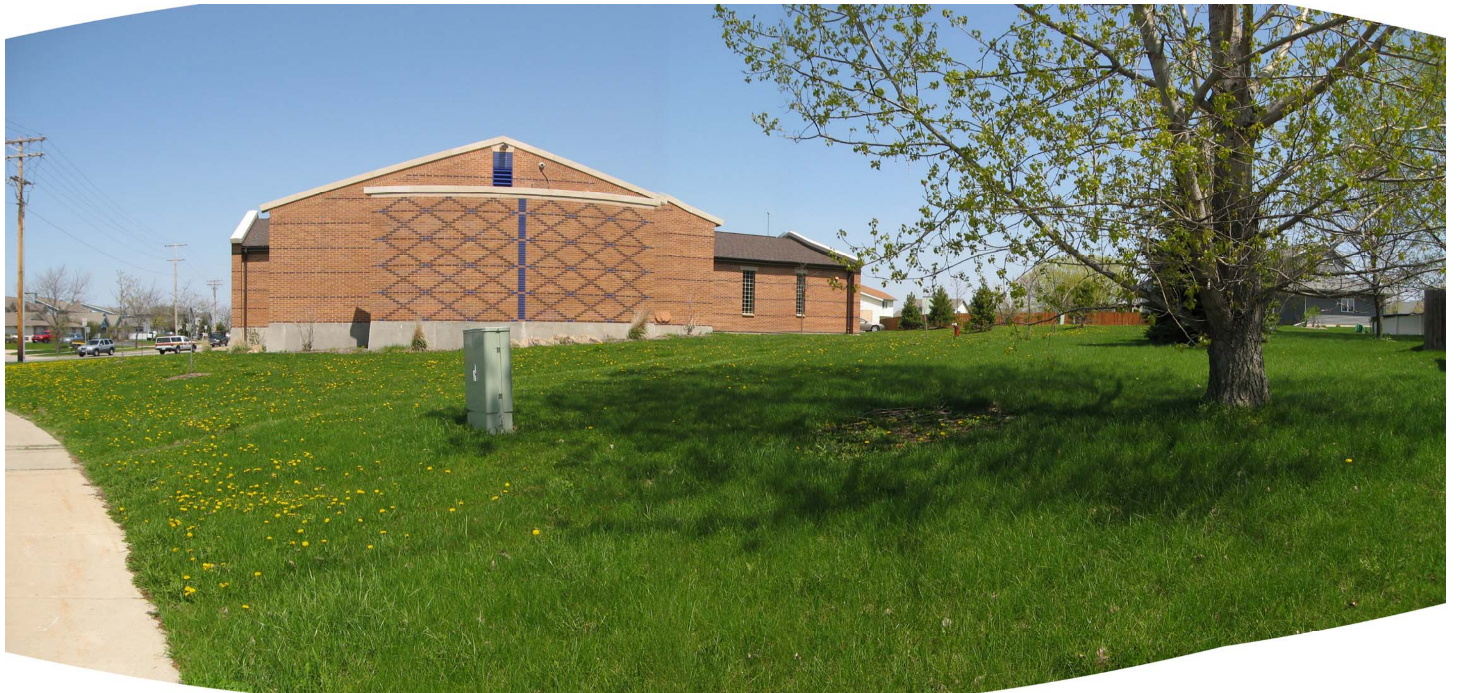
Photo: Madison Unit Well 29 Existing Facilities South property boundary looking north
