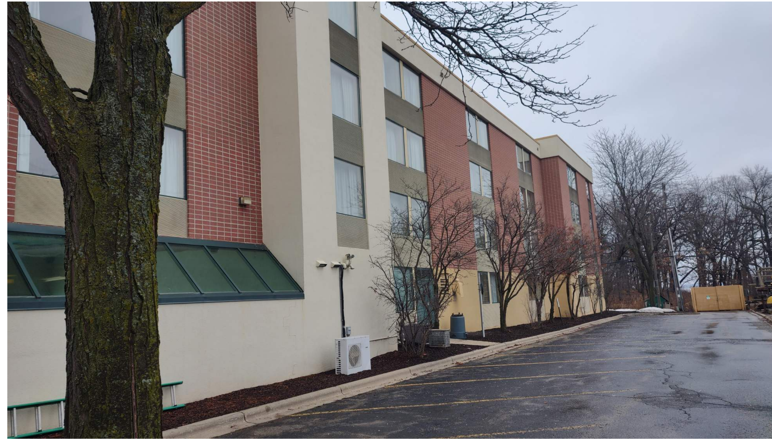
Existing Building Looking North
