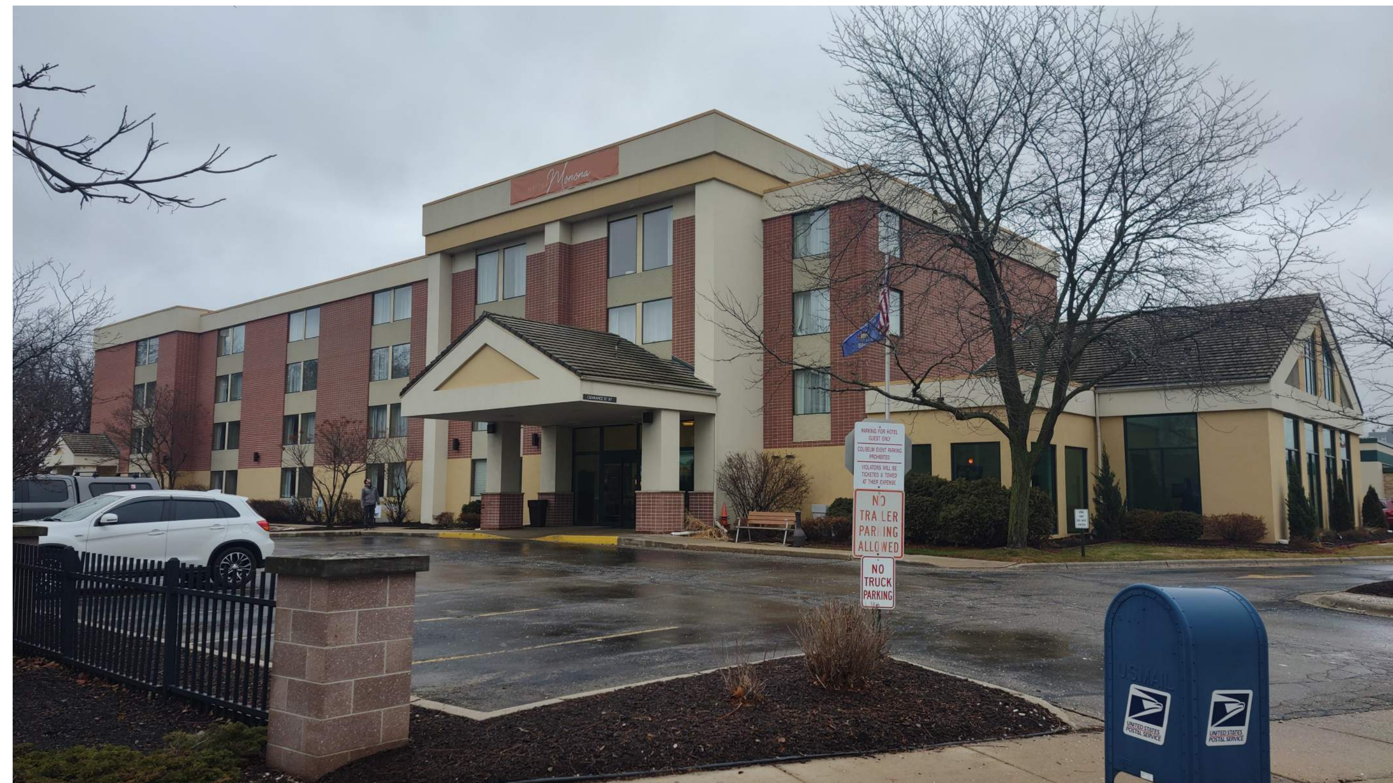
Existing Building Looking East
