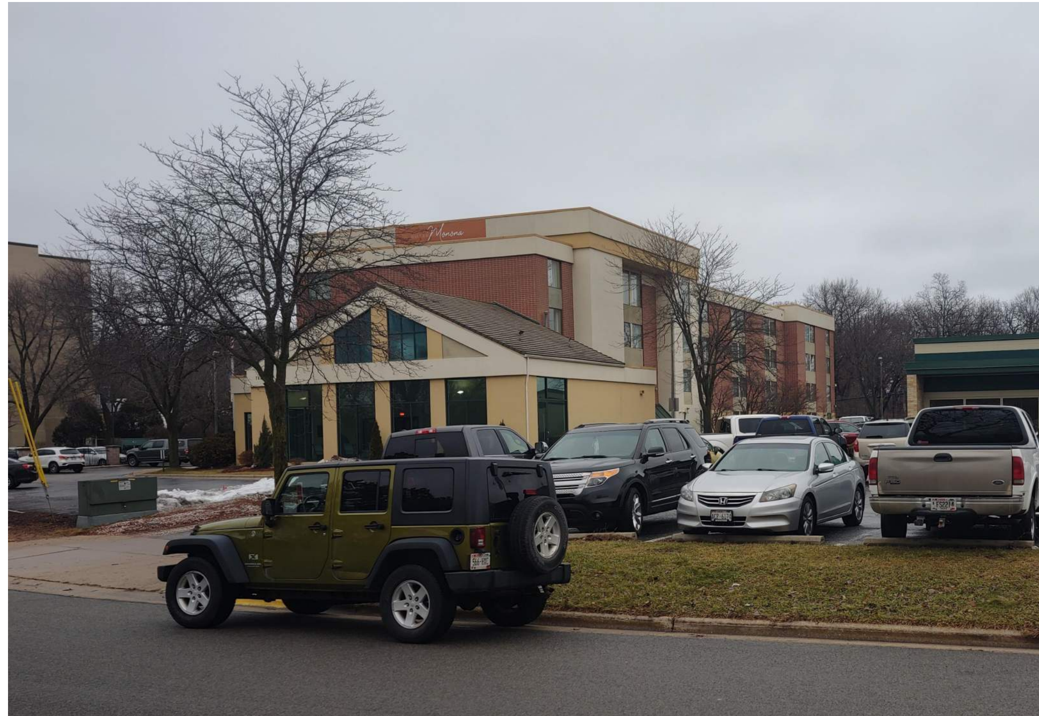
Existing Building Looking North
