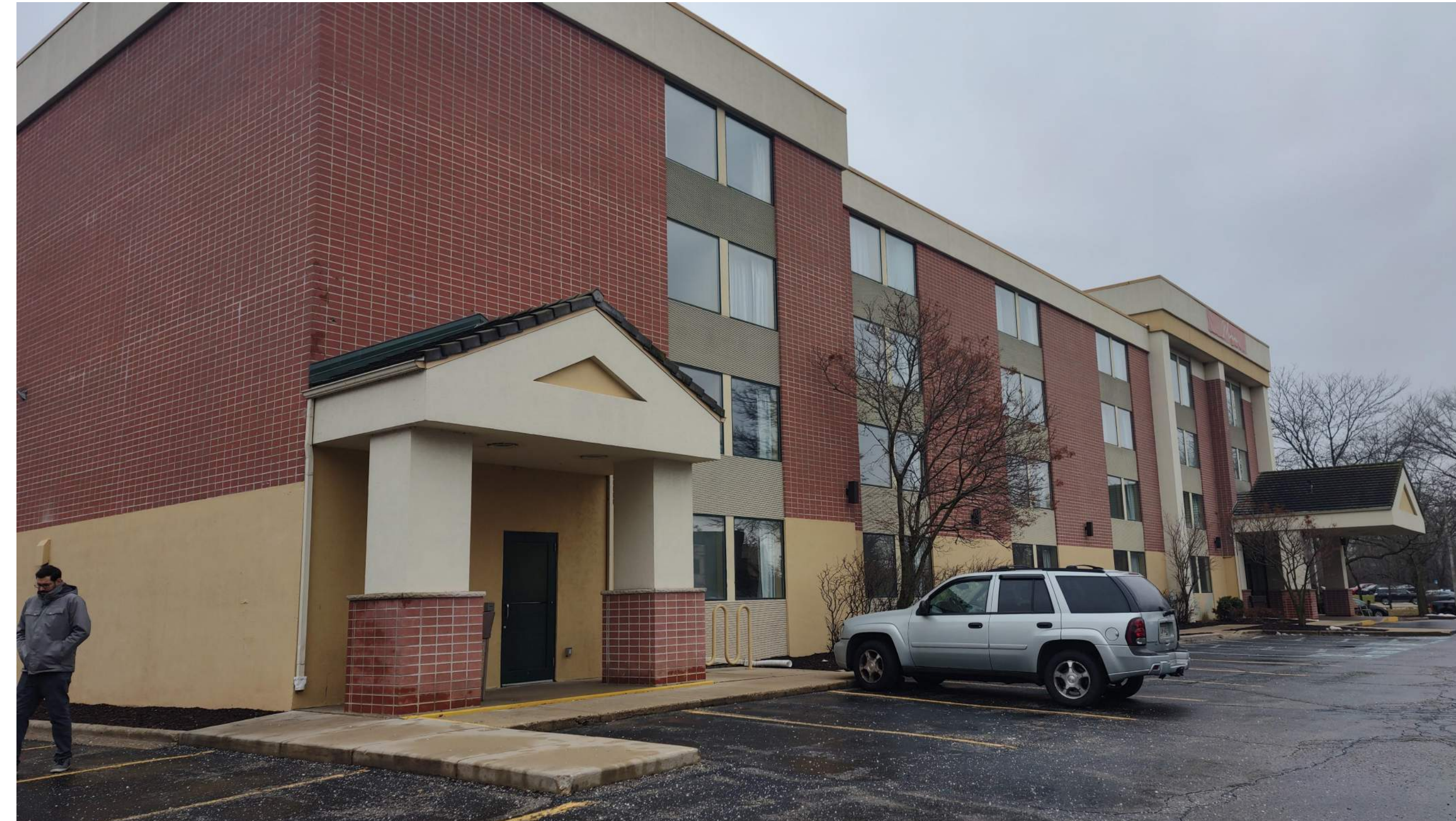
Existing Building Looking South
