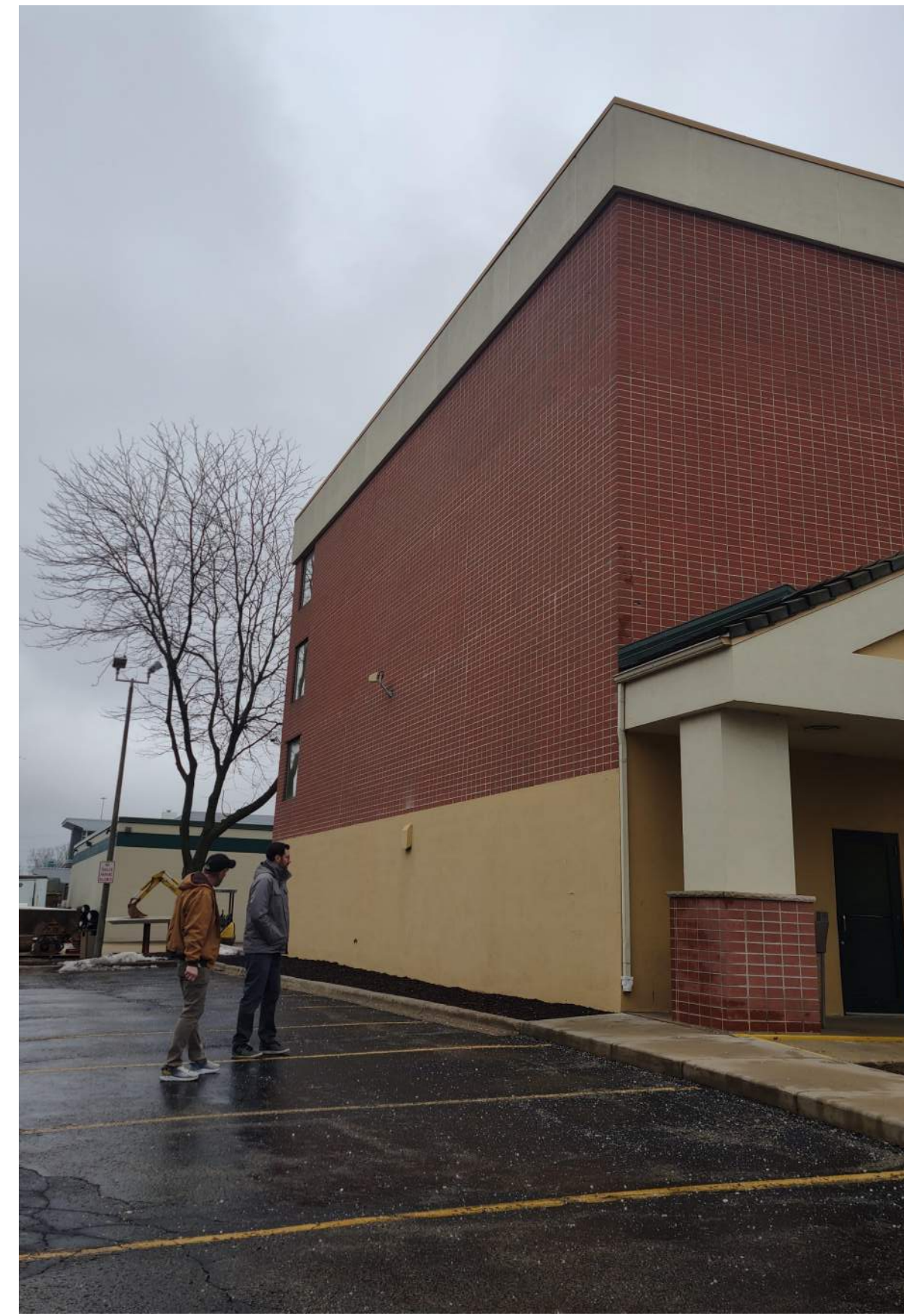
Existing Building Looking West
