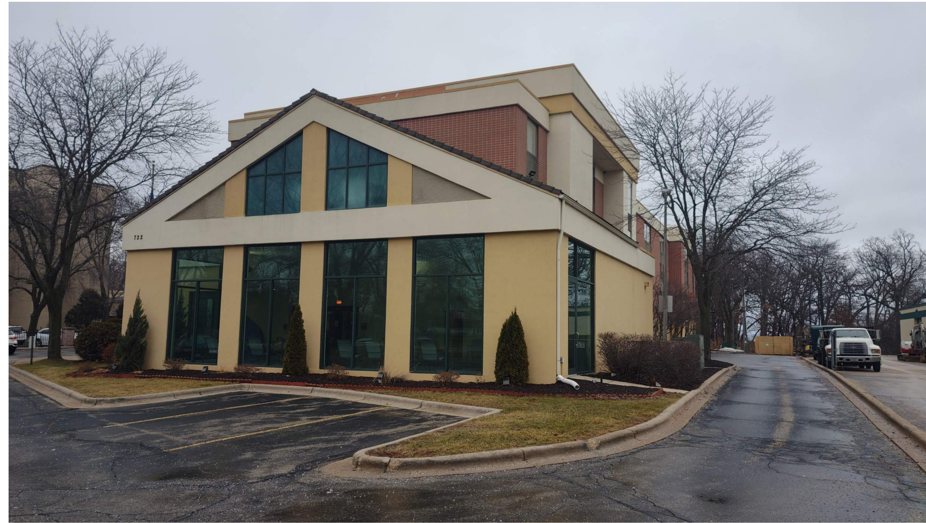
Existing Building Looking North
