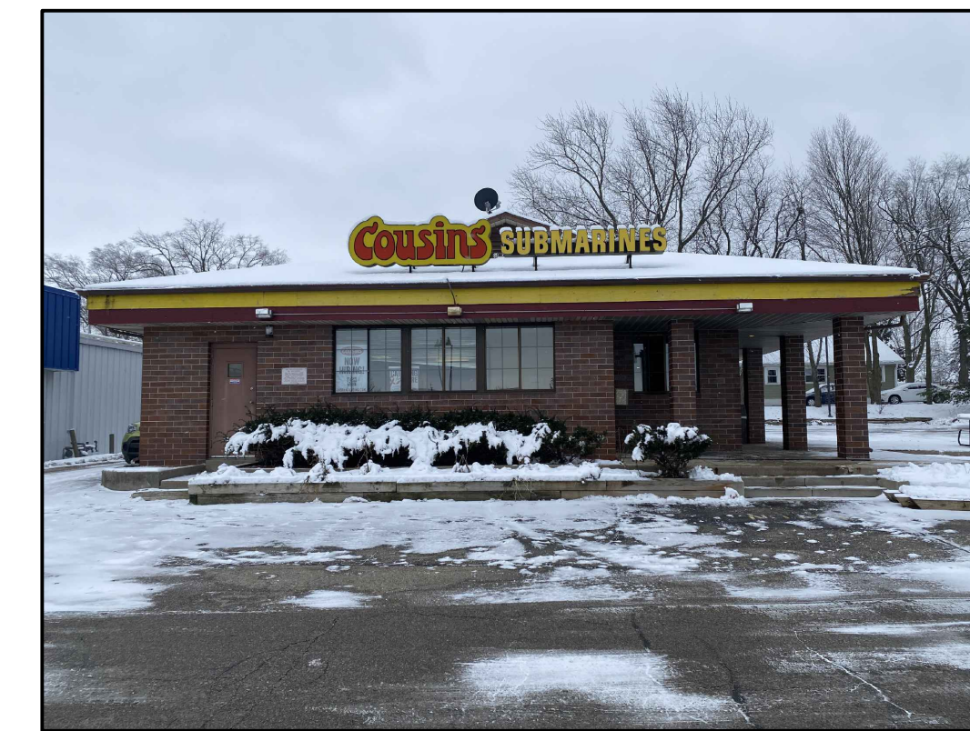
1 EXIST. NORTH PHOTO N.T.S.
