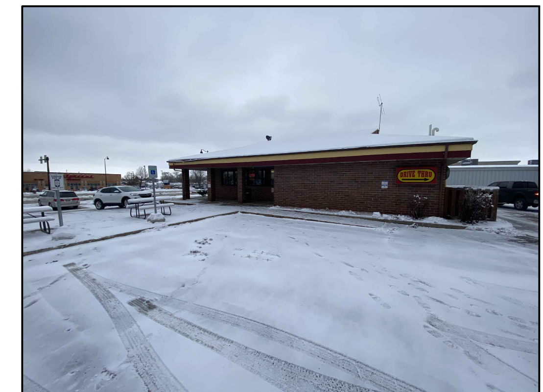
4 EXIST. WEST PHOTO N.T.S.
