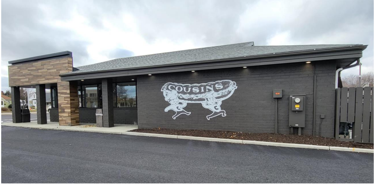
Photo #3 of completed remodel.
