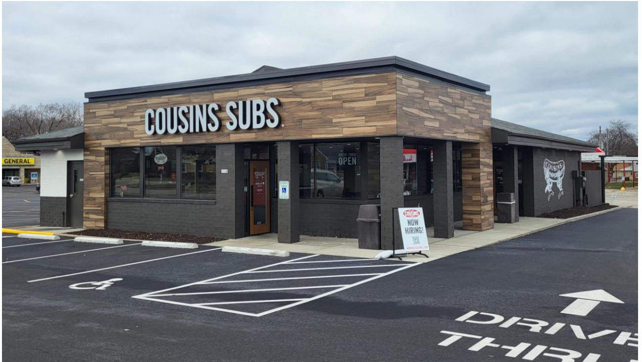
Photo #2 of completed remodel.
