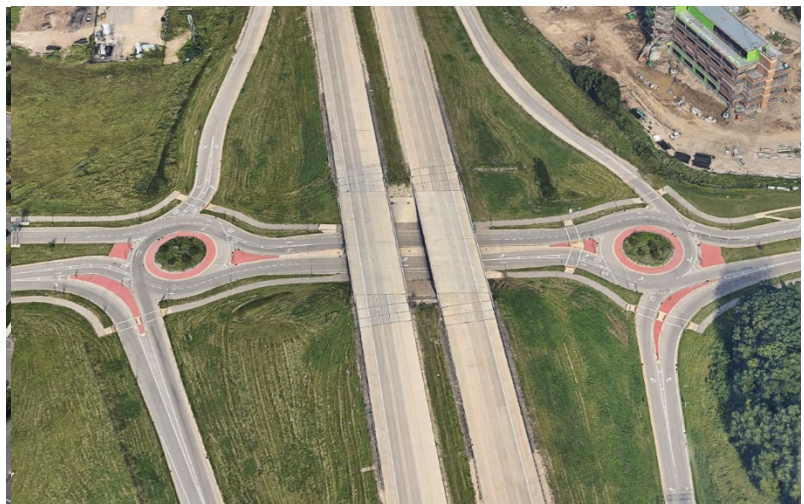
Functionally Concept 5 would operate in a similar manner to the County N interchange in Cottage Grove
