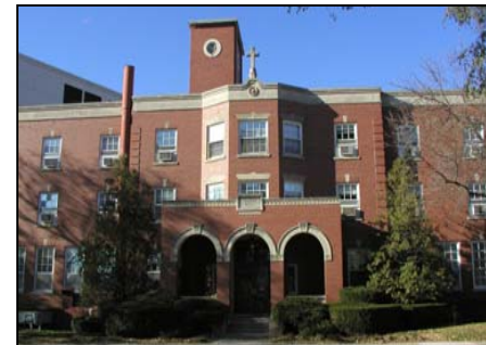
The former Longfellow School, now used as offices, is one of the most architecturally distinguished of all Madison's school buildings.
