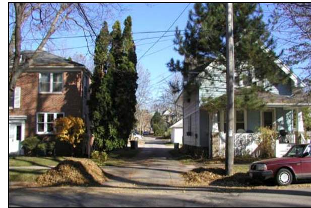
A typical neighborhood alley shown here separating residences near St. James Church.
