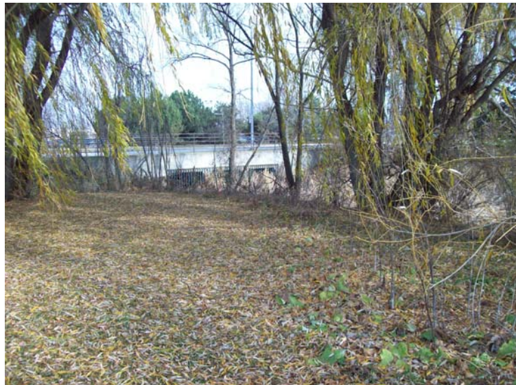
4. Looking northeast at the existing creek as it passes under Anderson Street. This will not be disturbed.
