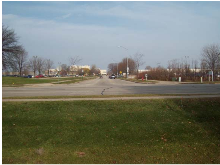
2. Looking north across Anderson Street down Hoffman Street. This would be where the extension of Hoffman would begin.
