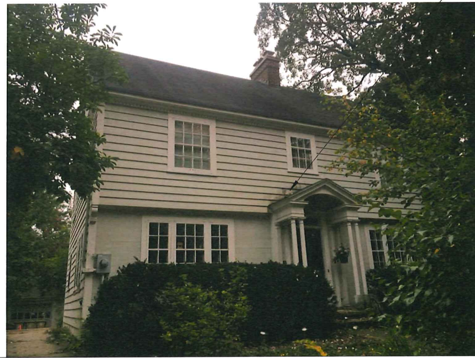
EXPOSED WOOD & CUPPING SIDING
