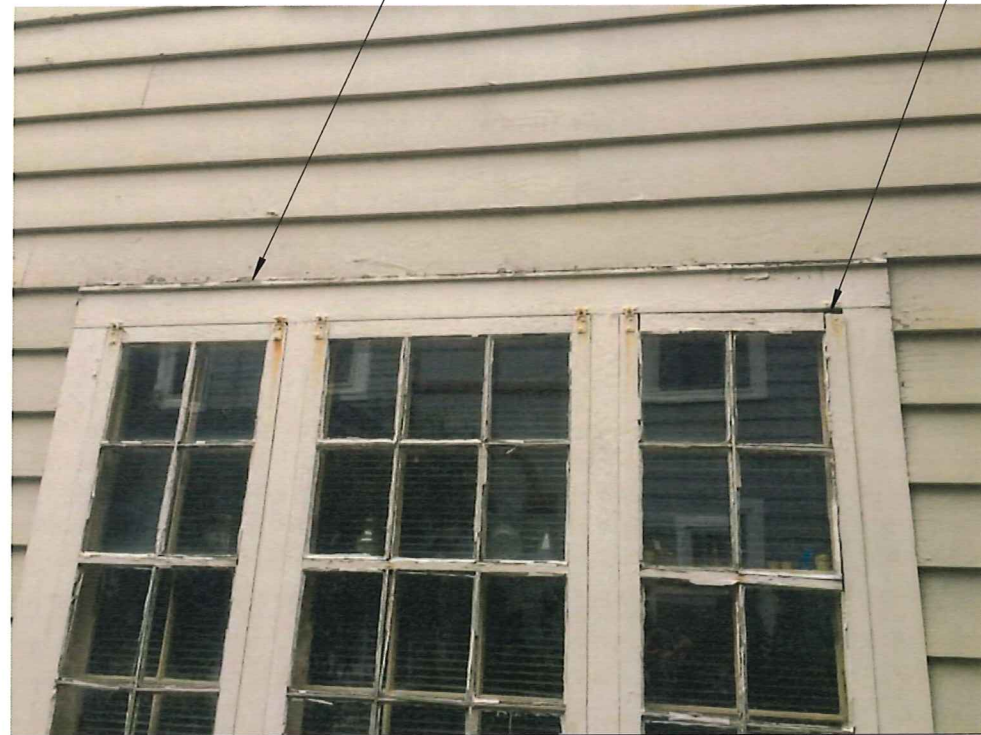
INSUFFICIENT GAP AT HEAD FLASHING
