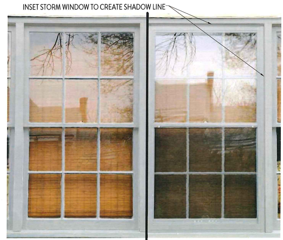
ORIGINAL WINDOW W/ NO STORM WINDOW (EXISTING STORM WINDOWS ARE FLUSH WITH MULLION) ORIGINAL WINDOW W/ NEW STORM WINDOW
