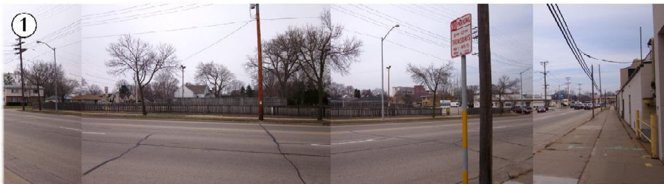
View Looking West From Fish Hatchery Rd.
