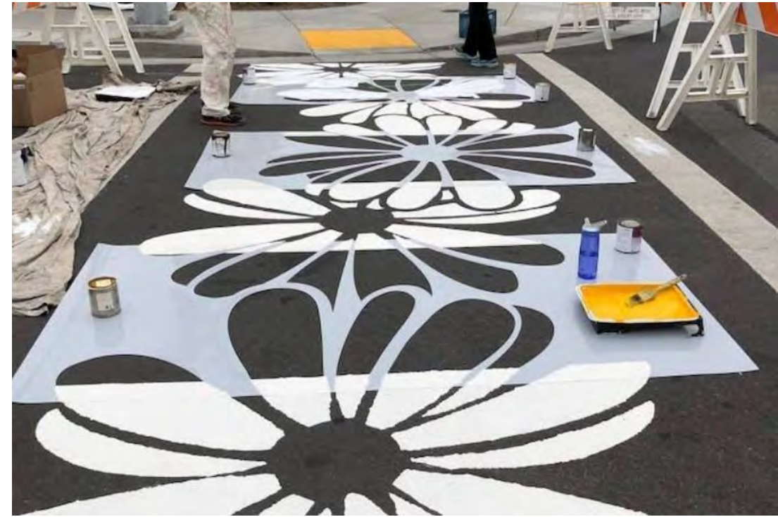
Street painting with slip resistant paint
