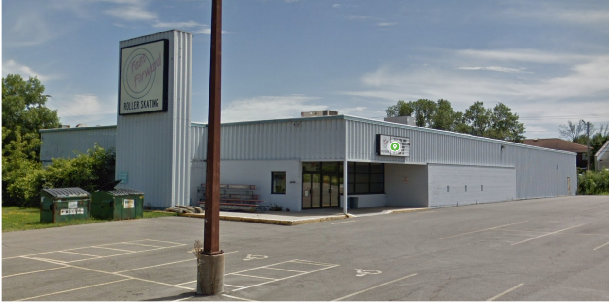
Southeast view of building
