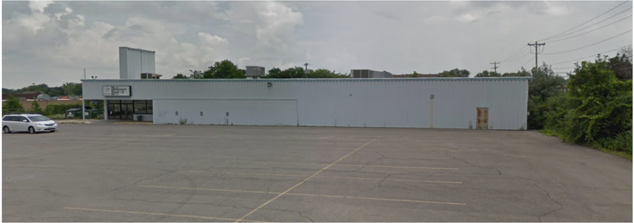
East side of building
