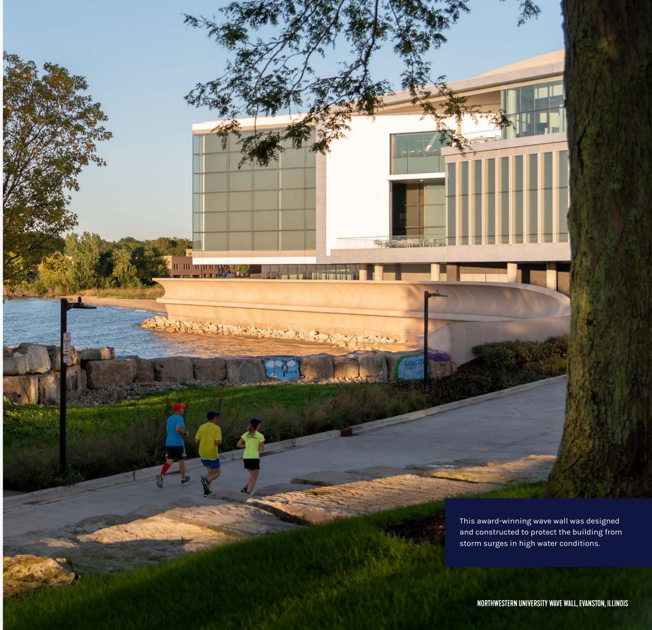
This award-winning wave wall was designed and constructed to protect the building from storm surges in high water conditions.
