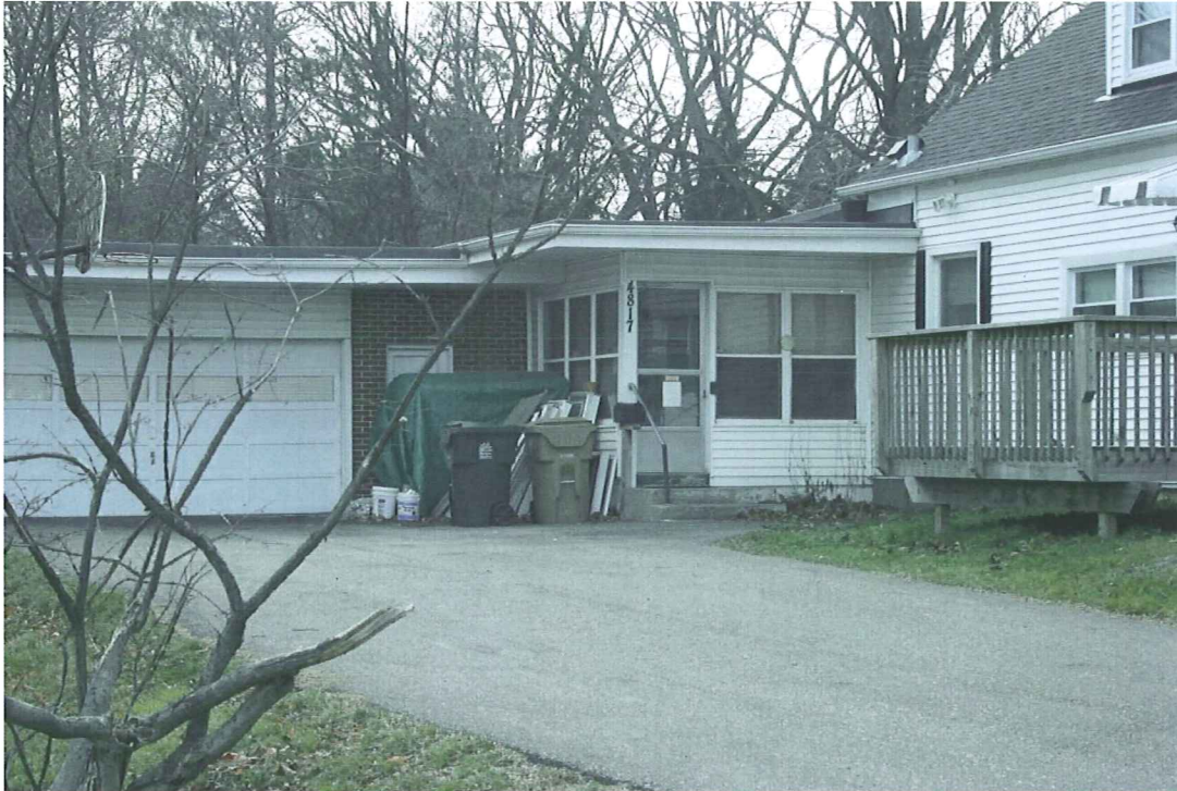
4817 Existing garage and three season porch
