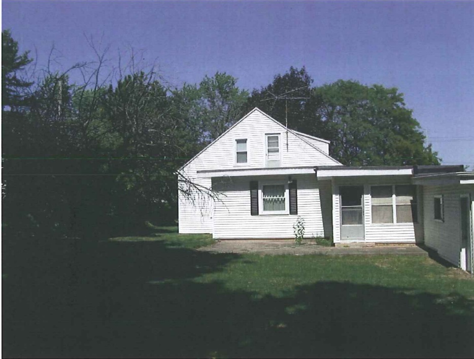
4817 North elevation of house
