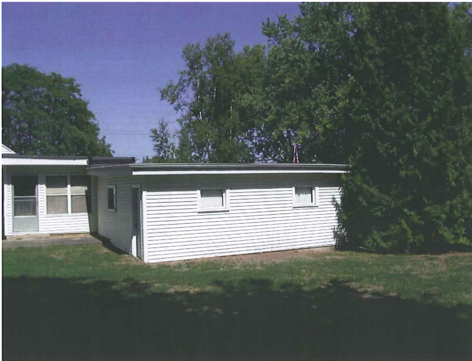
4817 North elevation of garage
