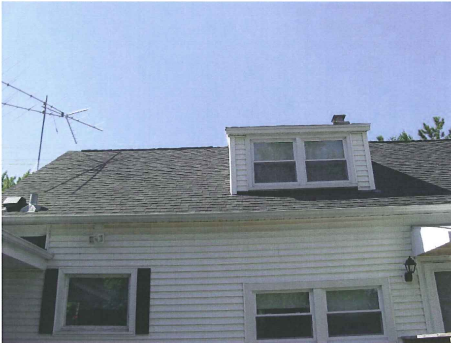
4817 Roof appears to be in good condition
