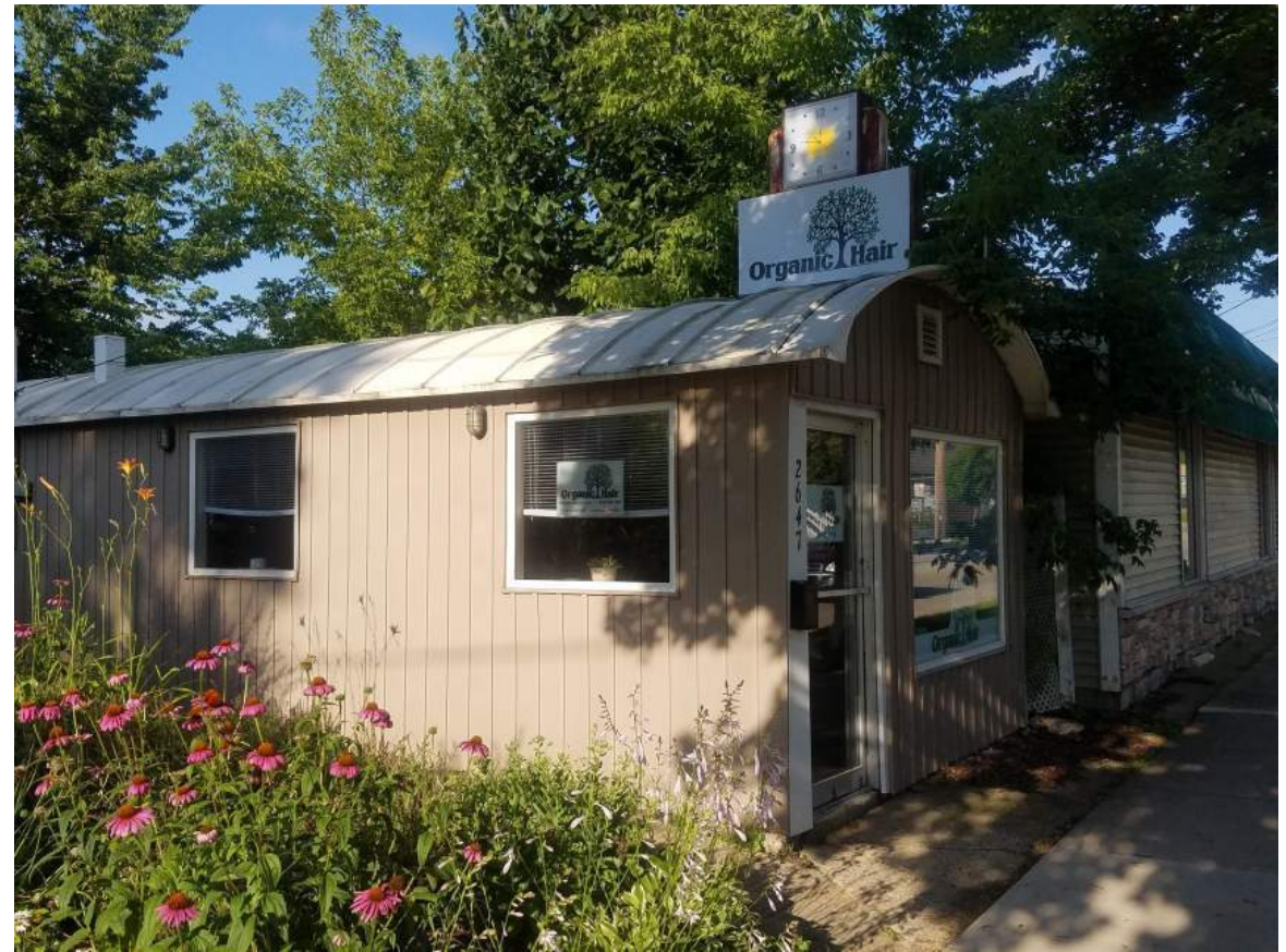
METAL QUONSET HUT TYPICAL EAST SIDE ECLECTIC AESTHETIC
