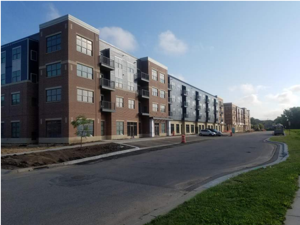
NEWLY BUILT APARTMENTS ACROSS WINNEBAGO FROM SITE LOOKING EAST
