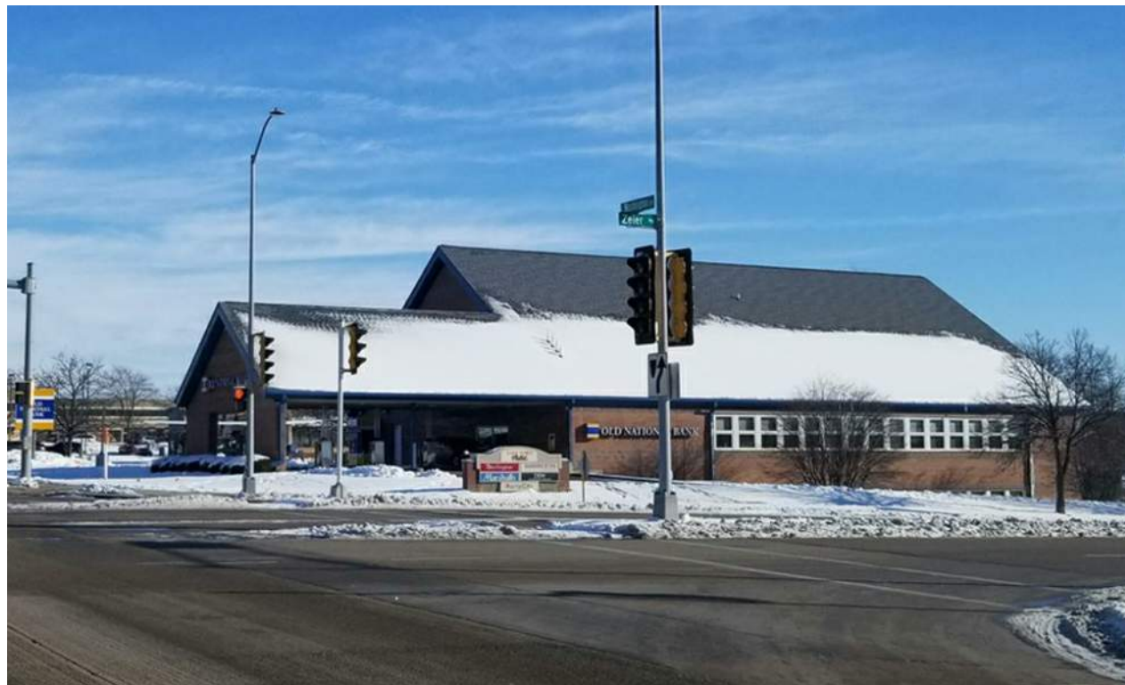
4702 EAST TOWNE BLVD - WEST ELEVATION
