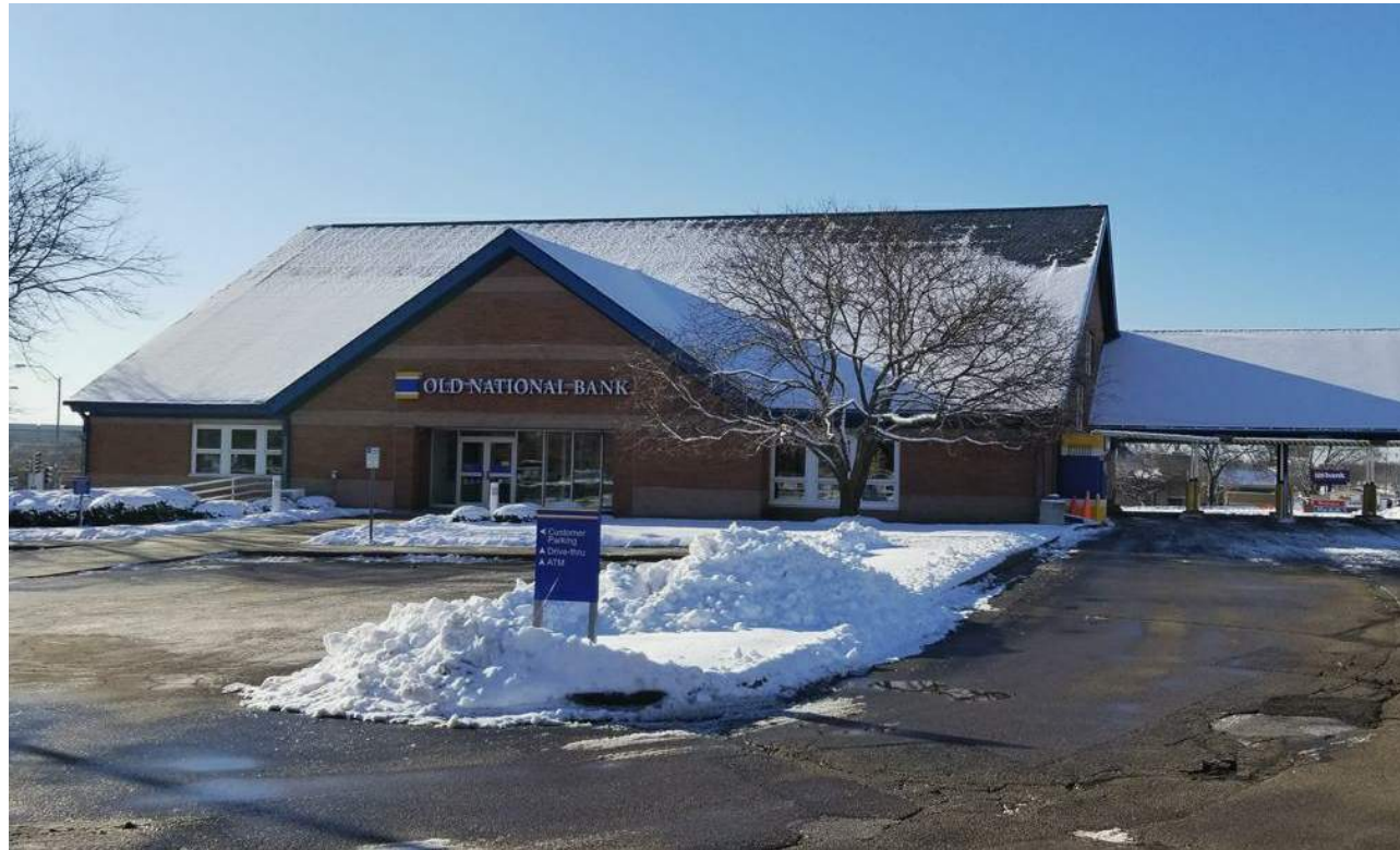
4702 EAST TOWNE BLVD - EAST ELEVATION
