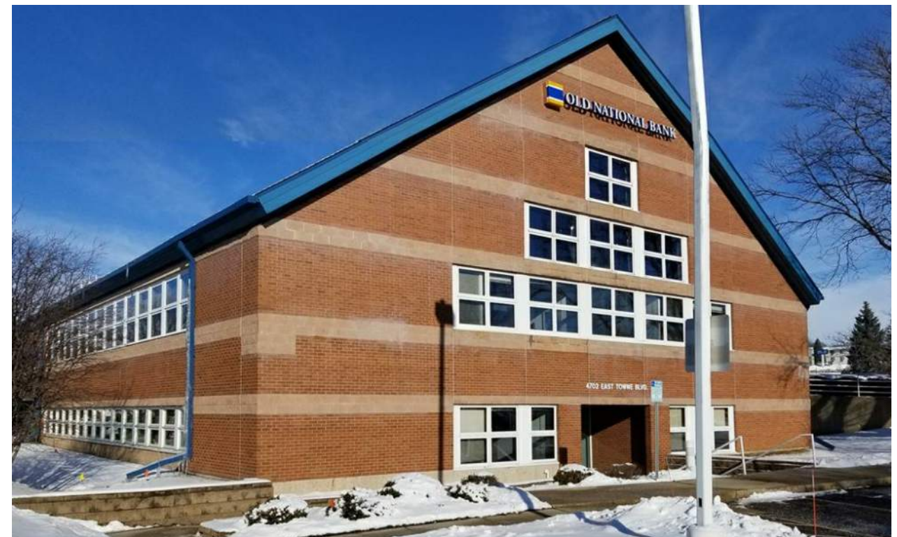
4702 EAST TOWNE BLVD - SOUTH ELEVATION
