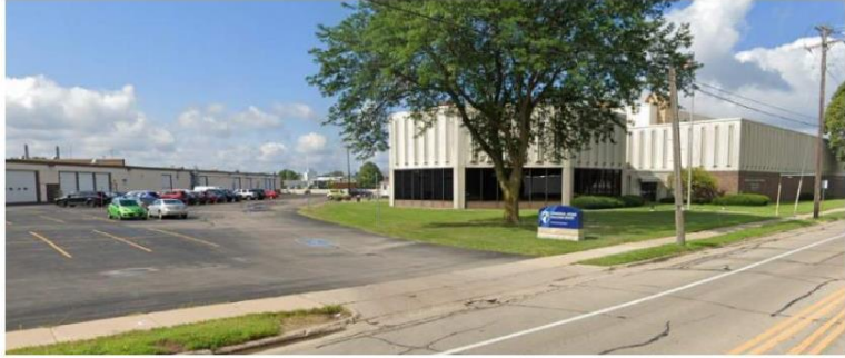
VIEW OF NEIGHBORING MADISON COLLEGE BUILDING A
