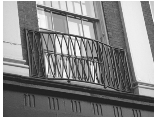
2 Painted Metal Railing Reference Image SCALE: N.T.S.
