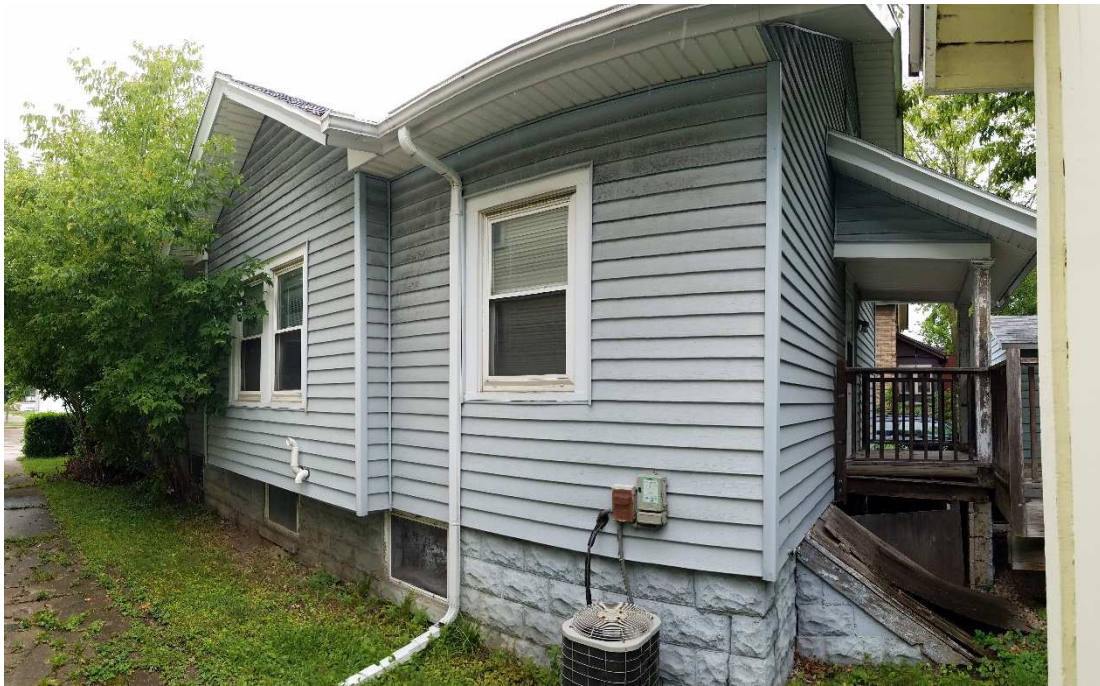
Exterior of 2305 E Washington Ave:
