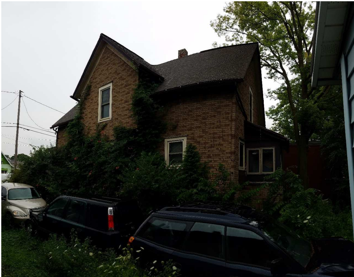
Exterior of 2311 E Washington Ave:
