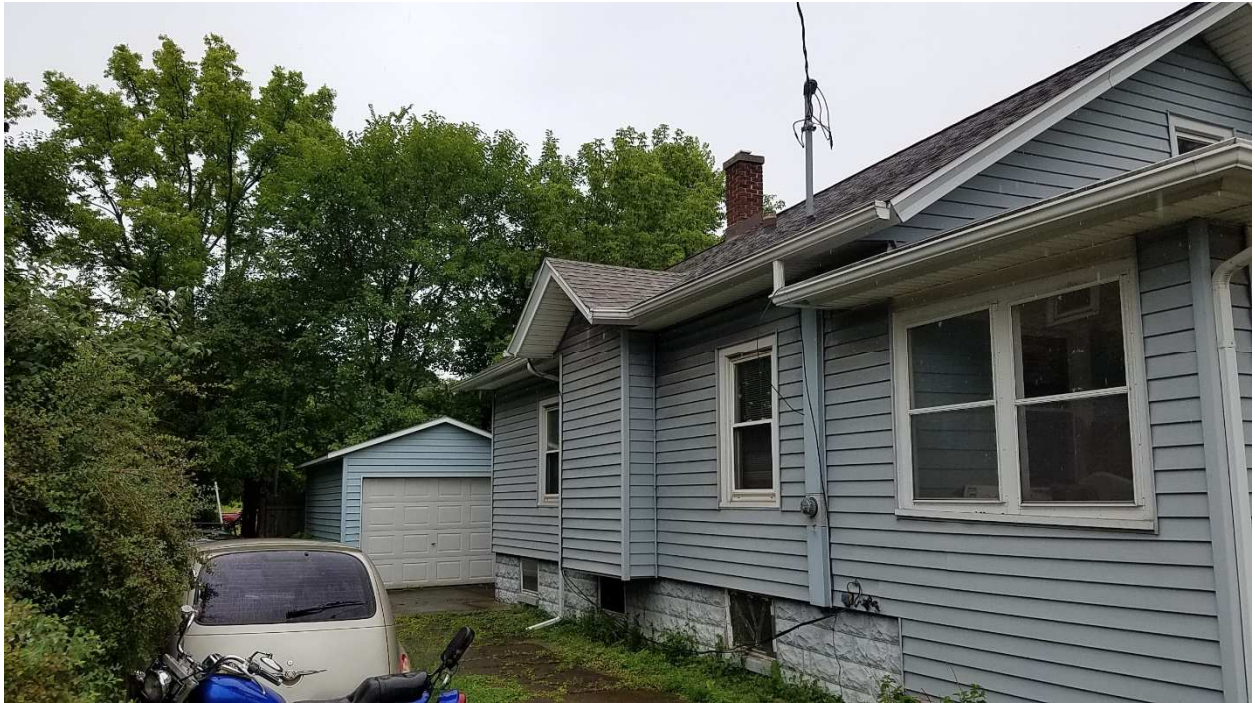
Exterior of 2305 E Washington Ave:
