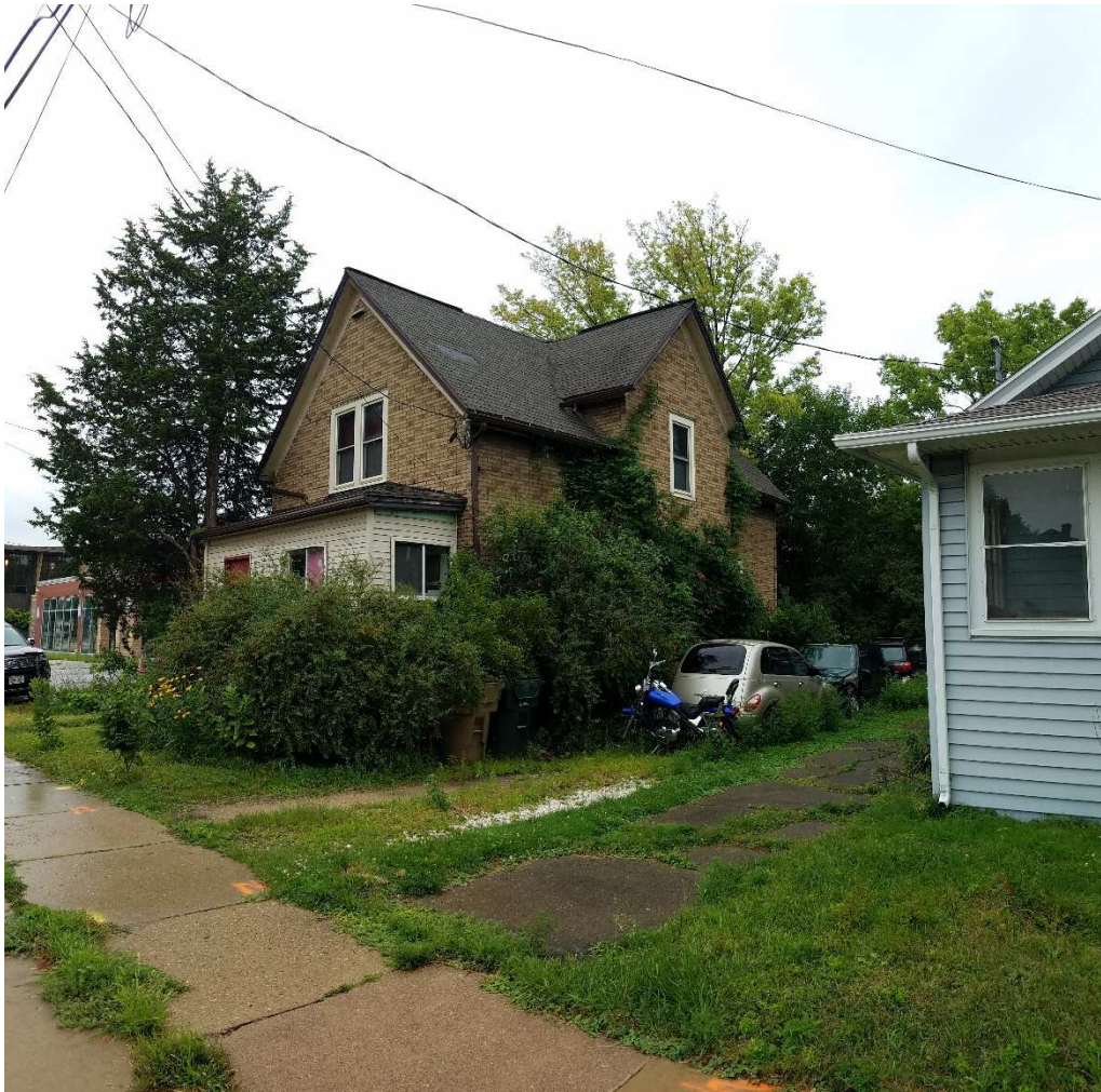
Exterior of 2311 E Washington Ave:
