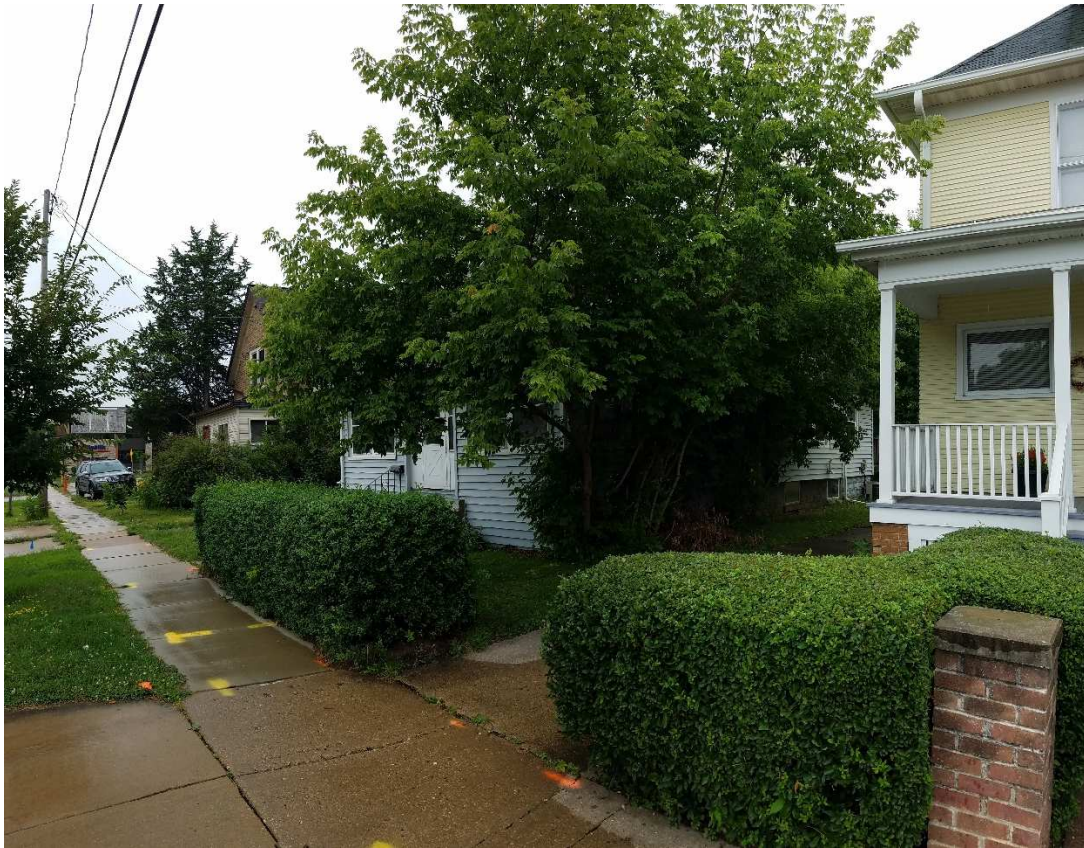
Exterior of 2305 E Washington Ave:
