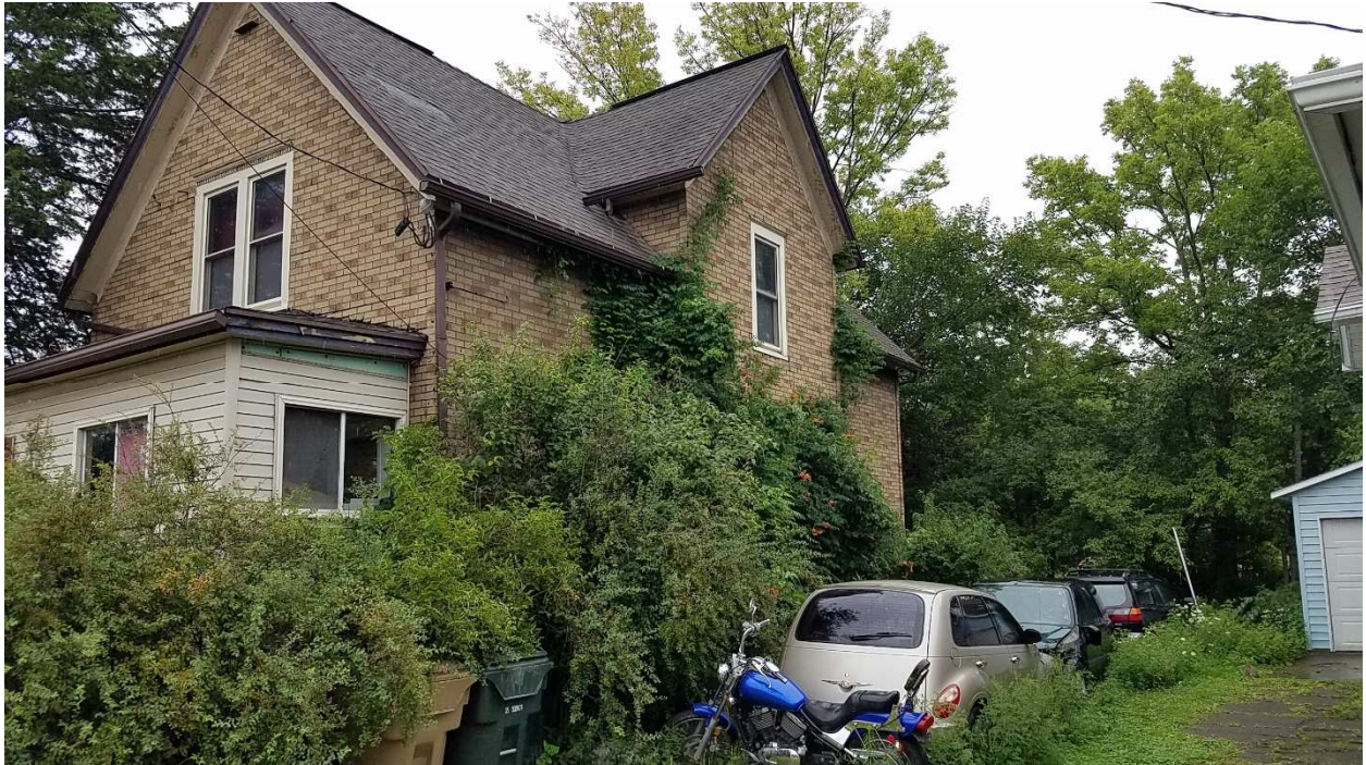
Exterior of 2311 E Washington Ave:
