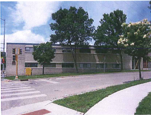
Exterior - East Elevation
