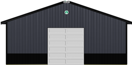
East End Wall 2 on Building 1
