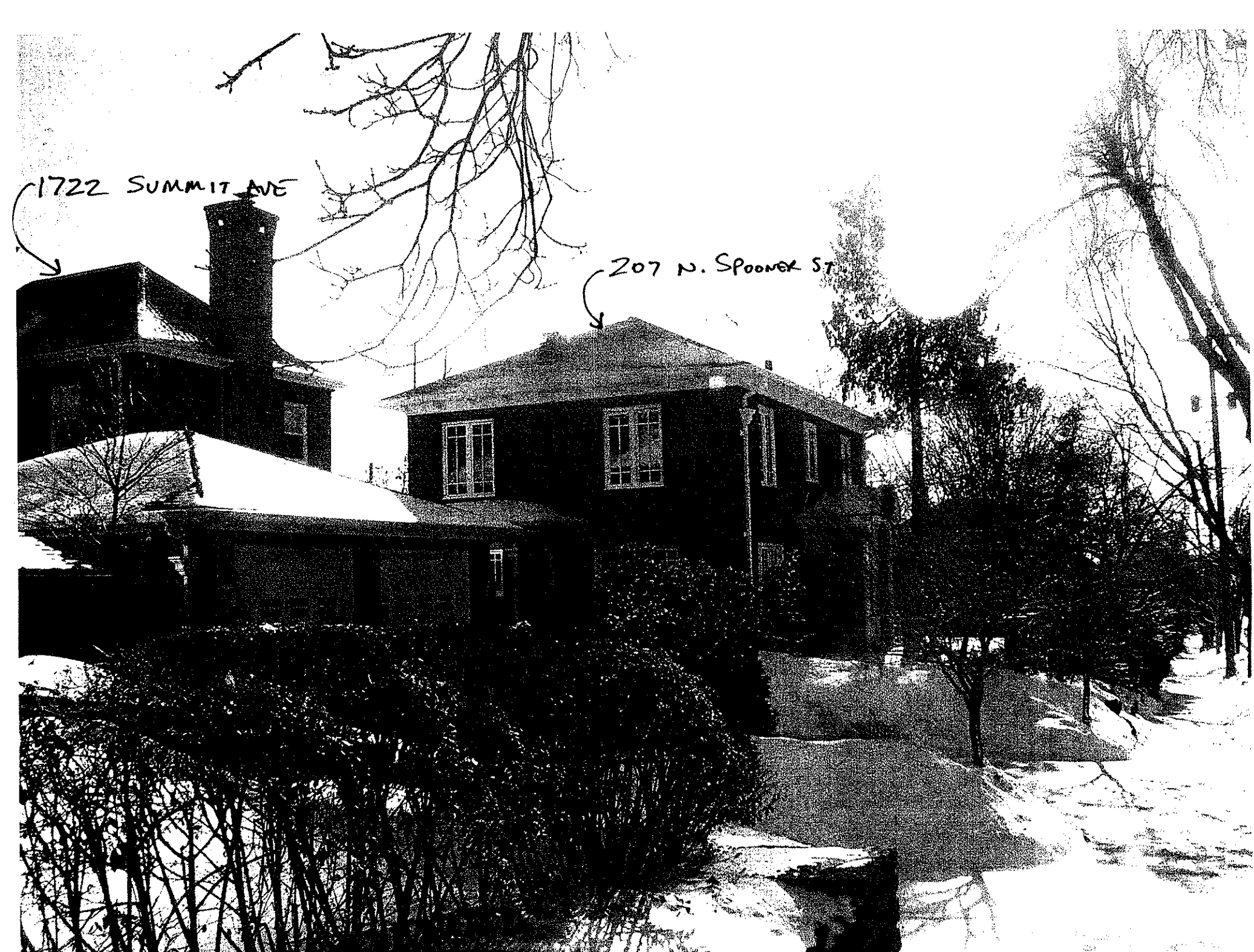
207 N. SPOONER ST EXISTING FACING SOUTH
