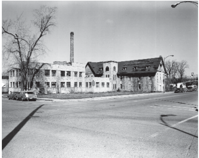
Abandoned Arcadian Springs Bottling Plant
