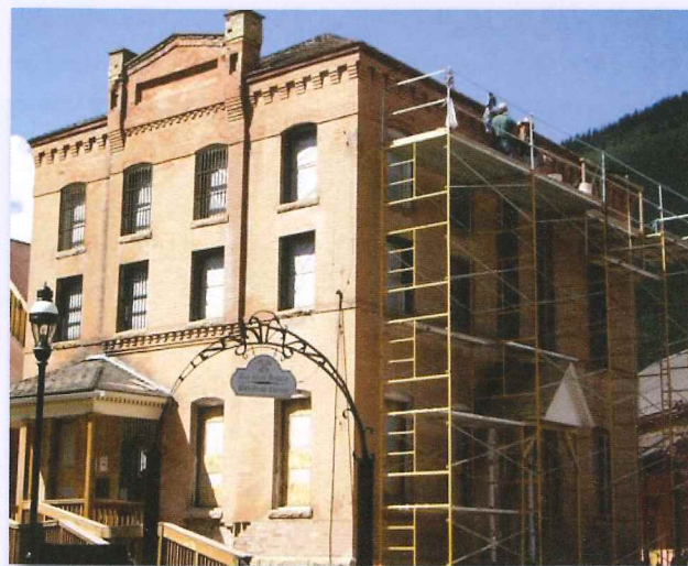
Top: Silverton Town Hall; Bottom: San Juan County jail building restoration
