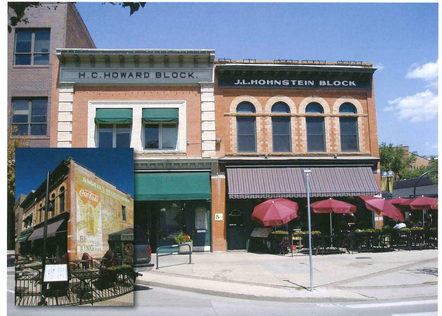
Historic Old Town Fort Collins has transformed into a thriving commercial district since historic district designation in 1979. Inset: A grant from the State Historical Fund will support the restoration of a historic Coca-Cola sign in Old Town Fort Collins.
