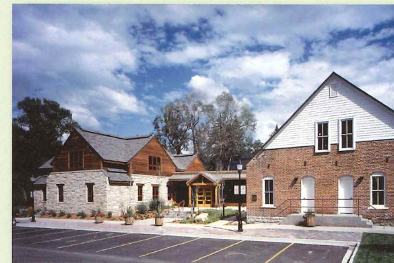
Centennial Hall-Carver Power Plant in Steamboat Springs (photo courtesy of John Robledo)
