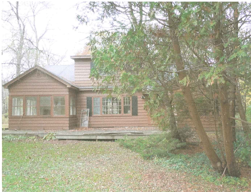
Lake side of that house. Clearance in the crawl space was only eighteen inches. House was raised five feet and placed on a new engineered flood resistant foundation. The work required a dewatering system as the water table was a foot below the yard and significant soil issues existed, requiring an engineered foundation based on a floating slab.
