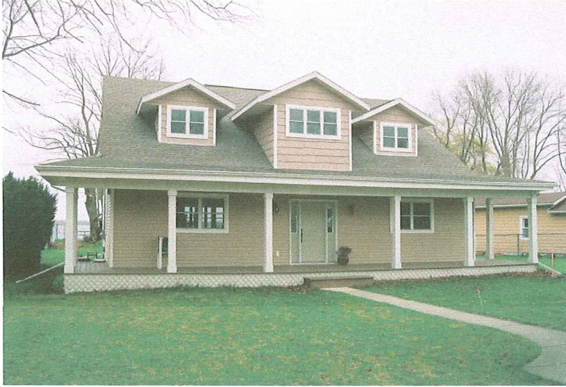
Front of 5908 Lake Edge, McFarland, a “pump and dump” project where the residential space was remodeled and the defective foundation left in place. The house was raised and placed on a new foundation.
