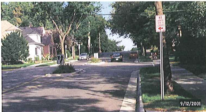
Typical parking restriction for a pedestrian refuge island (N. Baldwin St. at Mifflin St)
