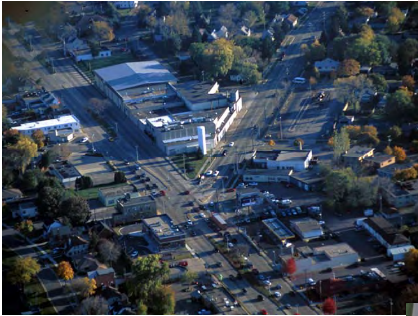
View of Dean/Morningstar Dairy site (looking south) at the intersection of South Park Street and Fish Hatchery Road. The building has been vacant since June 2004. Manufacturing equipment and other mechanicals have been removed from the building/site.
