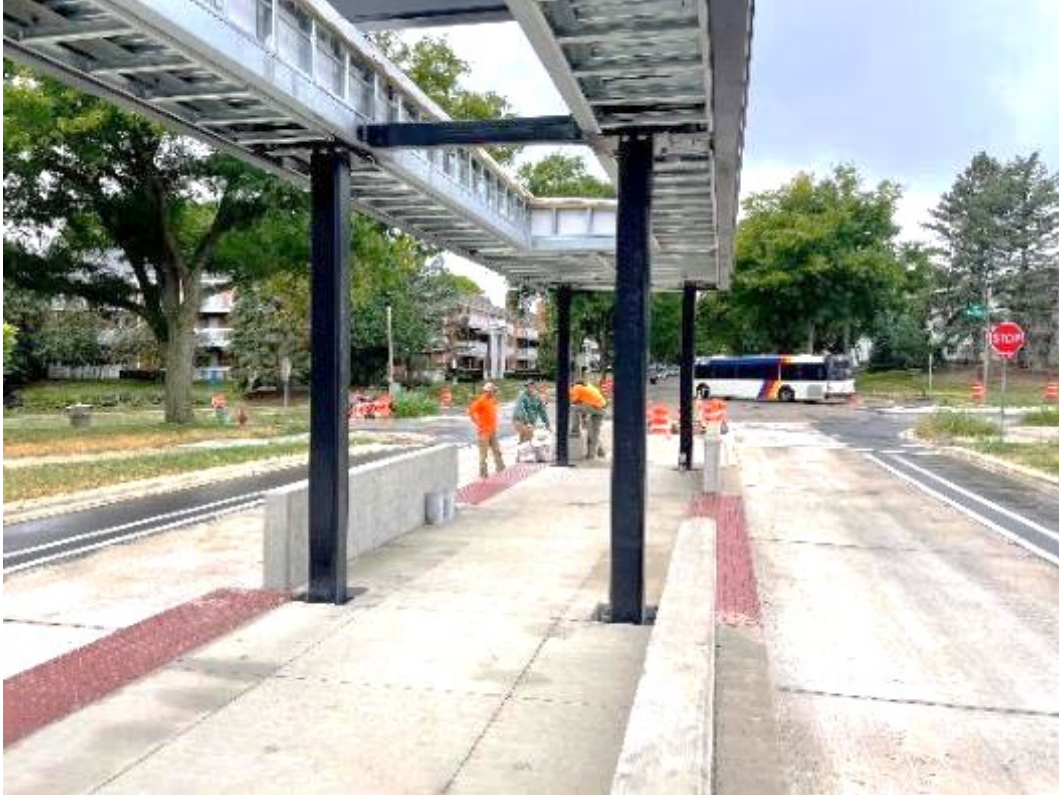
Figure 18 Eau Claire BRT Station Early Stages
