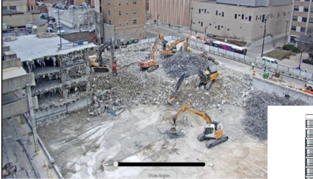
Figure 29 Demolition of State St Campus Garage Began in January 2024
