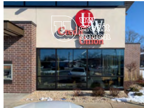
Remove existing sign and install new letters and logo Existing sign size 101" x 78"
