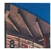
8. STAINED WOOD DECK AND BEAMS
