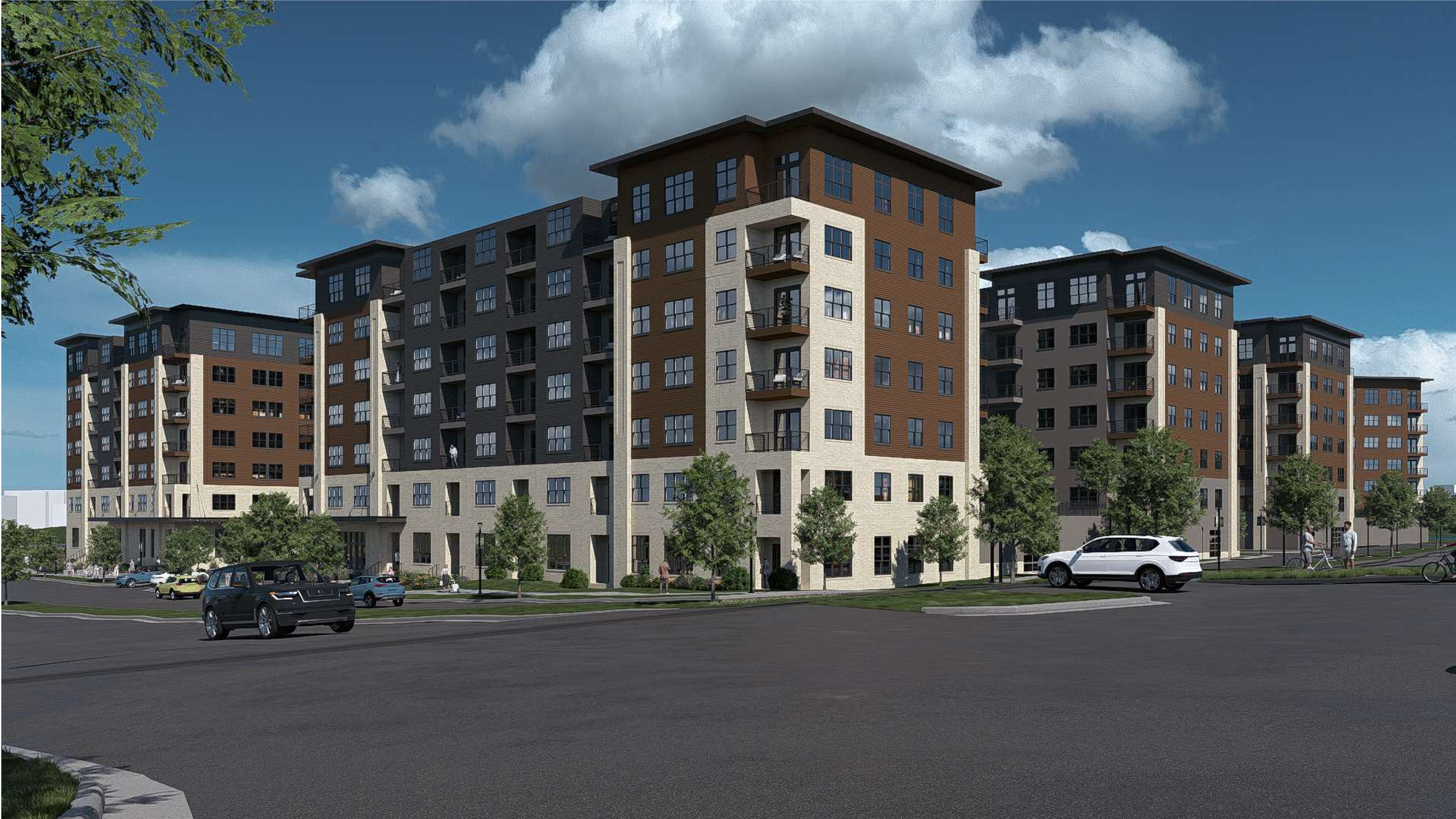
VIEW LOOKING NORTHEAST FROM WHITNEY WAY
