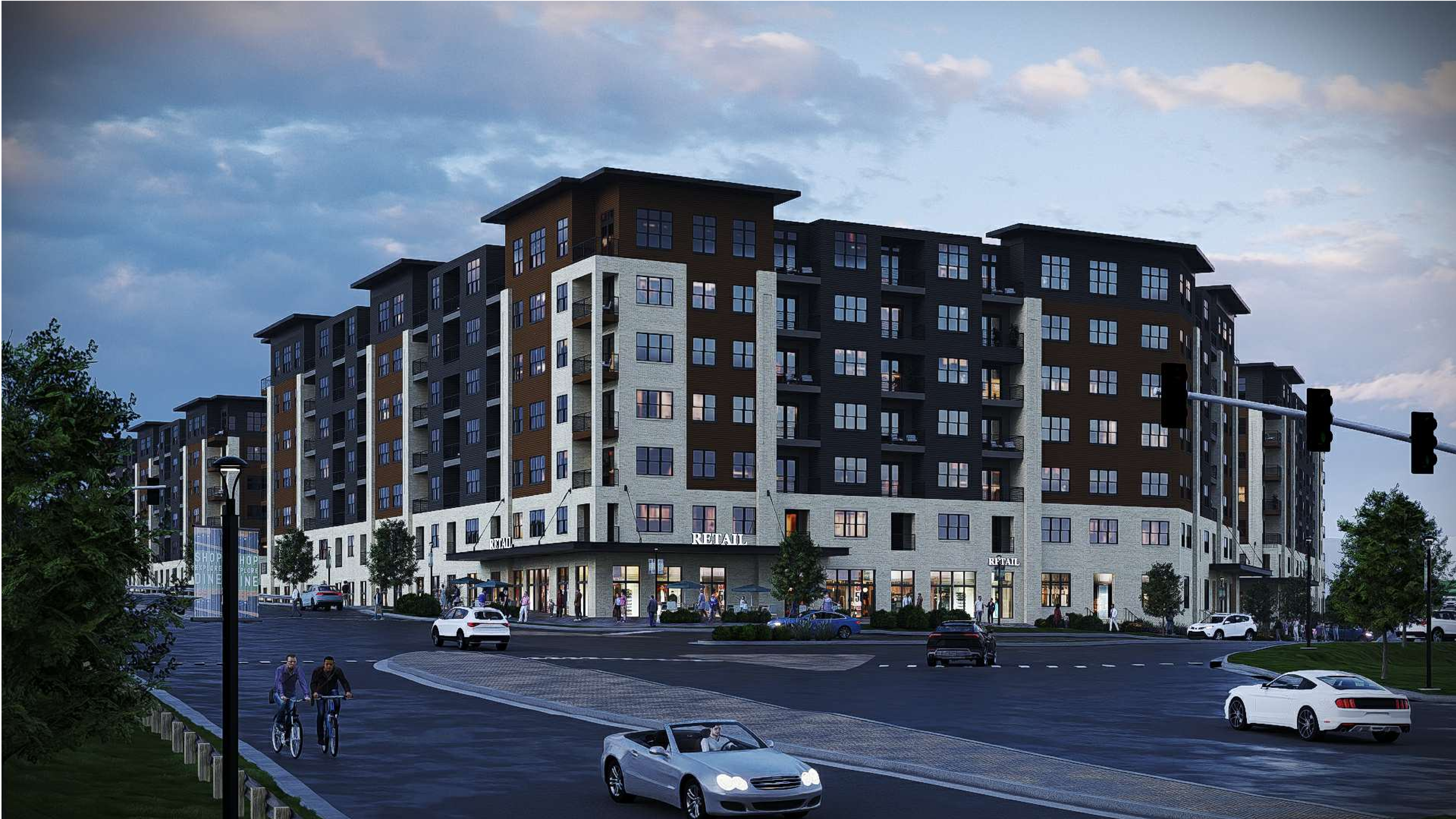
VIEW LOOKING SOUTHEAST FROM UNIVERSITY AVENUE
