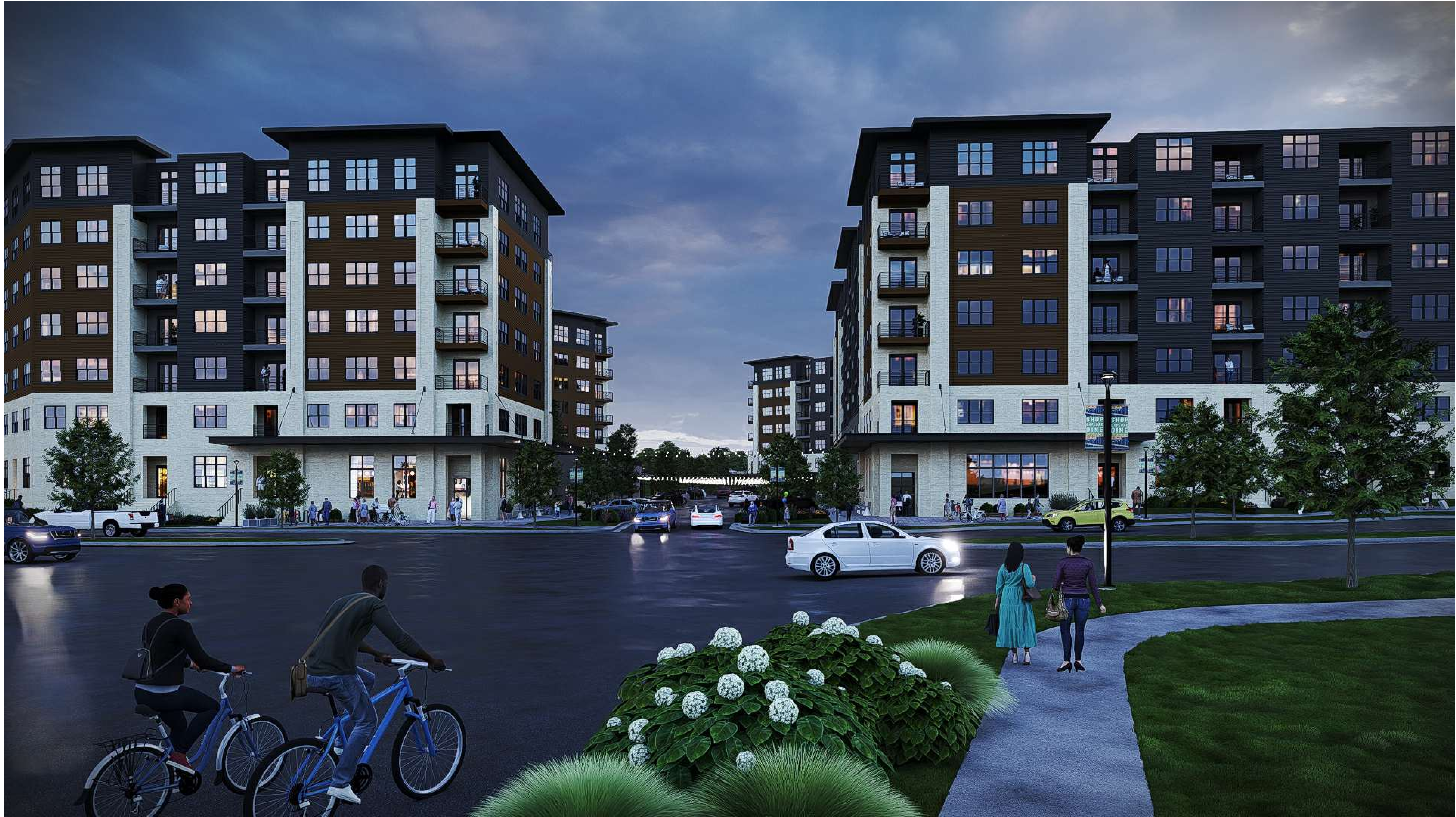
VIEW LOOKING EAST FROM WHITNEY WAY
