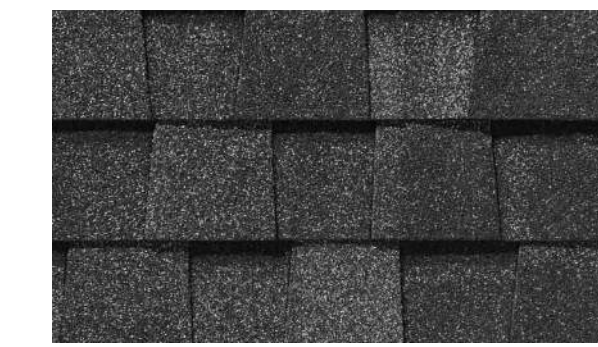
CERTAINTED ASPHALT SHINGLE ROOF - PEWTER
