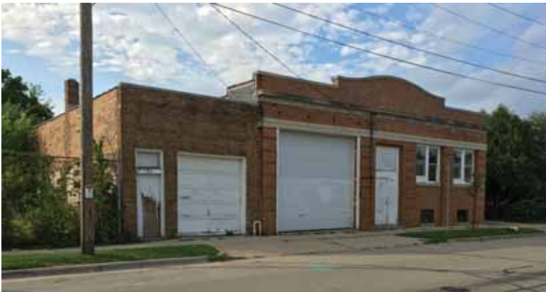
924 East Main St - To be Demolished
