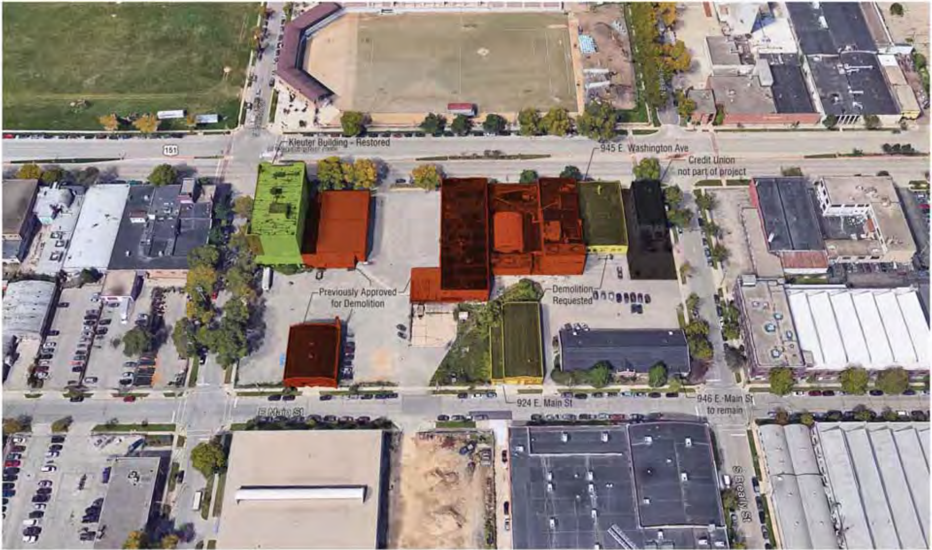
D1. Demolition Context Aerial Archipelago - Madison January 23, 2019
