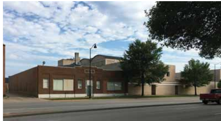
945 East Washington Ave - To be Demolished
