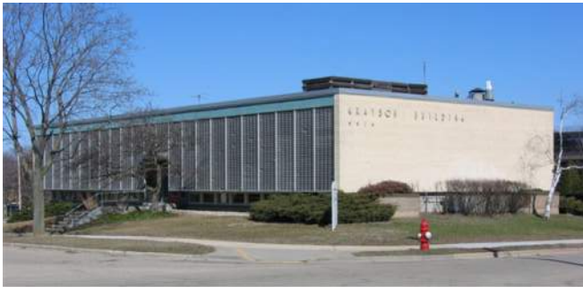
Grayson Building 4414 Regent Place
