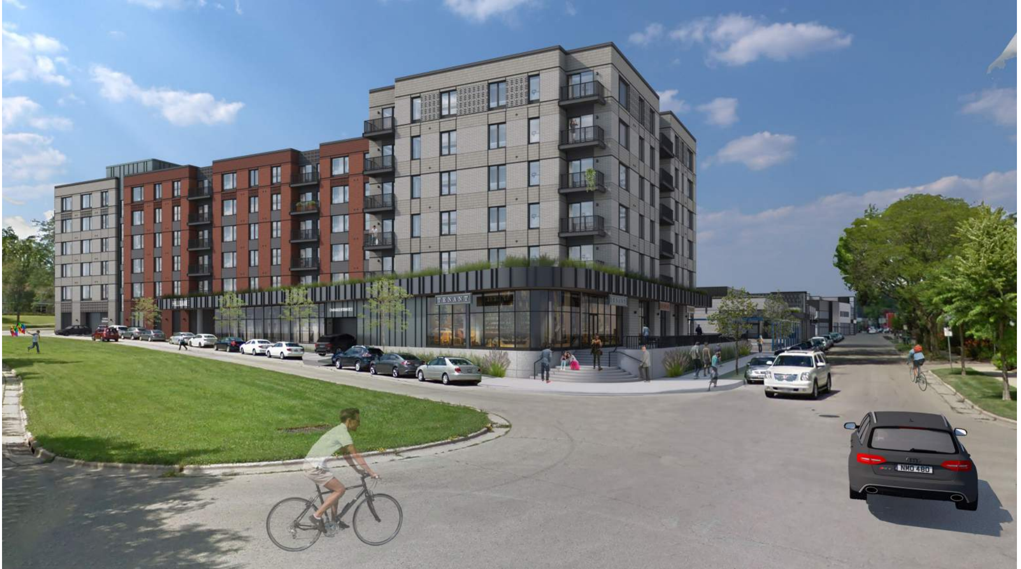
HILLDALE PHASE 3 View from Price Place at Vernon Blvd
