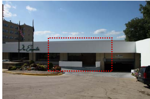
Figure 3.1 Current Loading Dock
