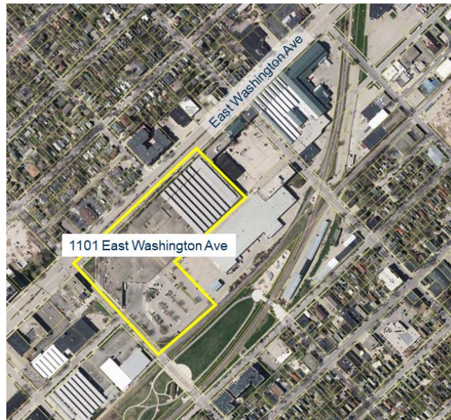
Figure 2.1-1 Existing 1101 East Washington Ave Facility
