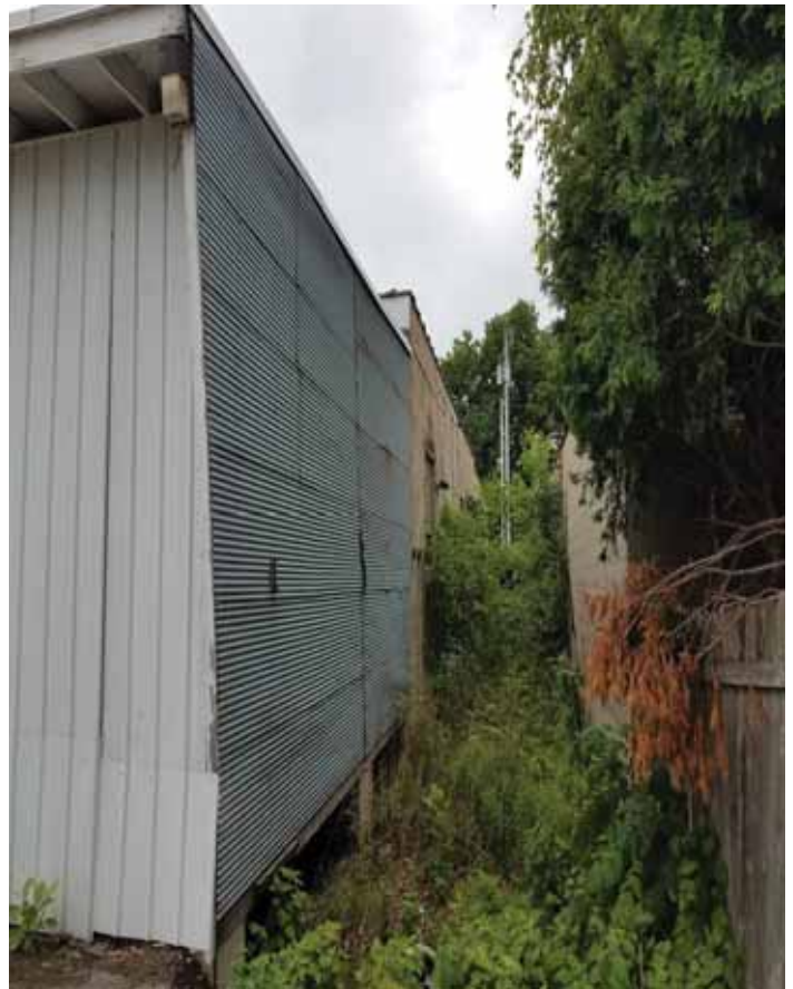
EXTERIOR OF NORTHEAST REAR OF RECEIVING AREA.
