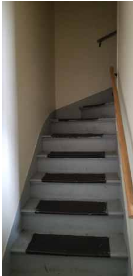
REAR ENTRY STAIR, ACCESS TO APT #3A, 3B & BASEMENT
