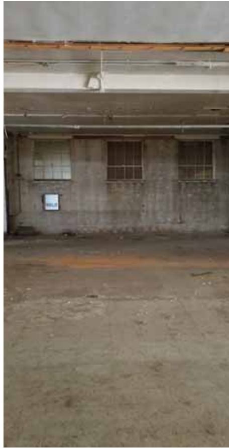
CENTRAL SPACE, MAIN FLOOR.
