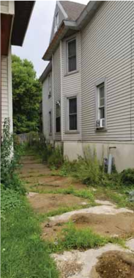
WEST SIDE OF APARTMENT.
