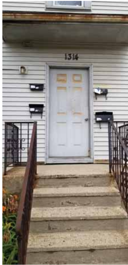
FRONT ENTRANCE, E WASHINGTON AVE.
