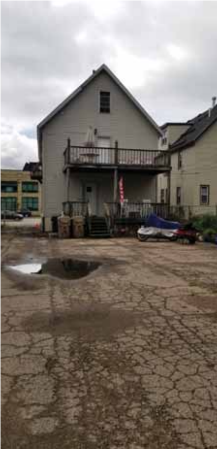
REAR OF APARTMENT.
