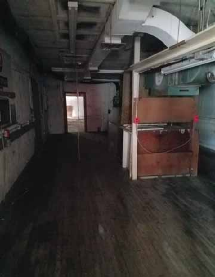
HALLWAY TO REAR SPACE (OPPOSITE BASEMENT STAIRWAY).
