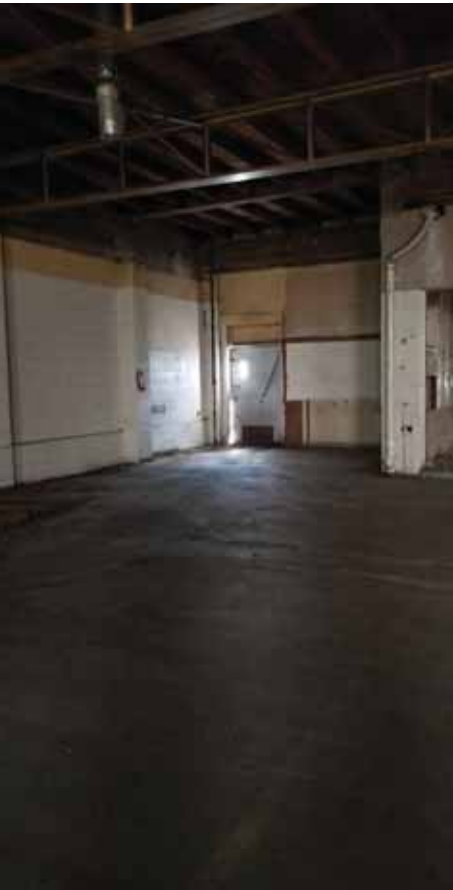
RECEIVING AREA, MAIN FLOOR.
