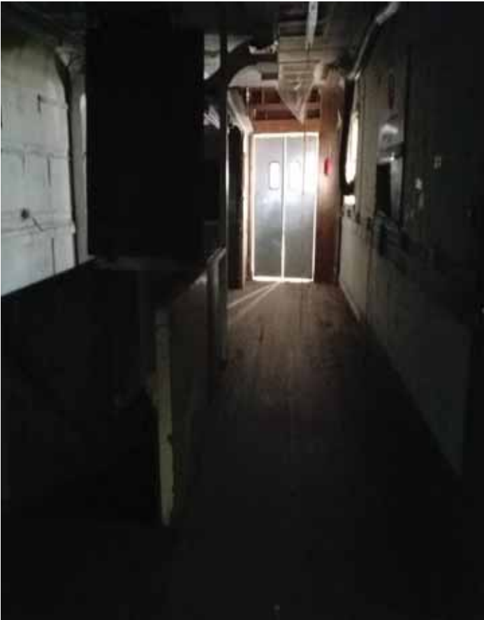
HALLWAY TO BASEMENT STAIRWAY (OPPOSITE REAR SPACE).
