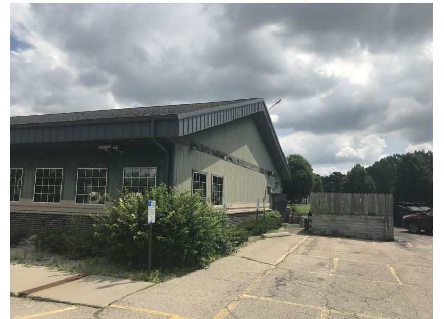
Existing Building South End - Looking to NE
