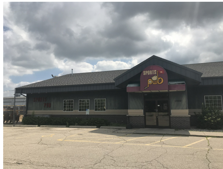
Existing Building West Entry - Looking to NE
