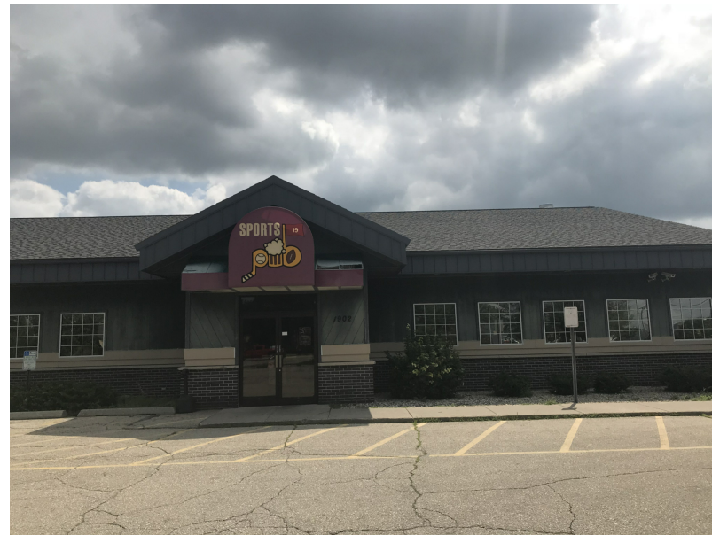
Existing Building West Entry - Looking to E
