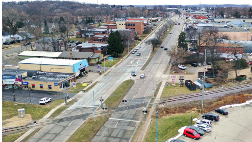
An aerial photo of the South Park Street corridor. Last year, the city purchased property at 1810 S. Park St. for land banking purposes. PHIL BRINKMAN, STATE JOURNAL
