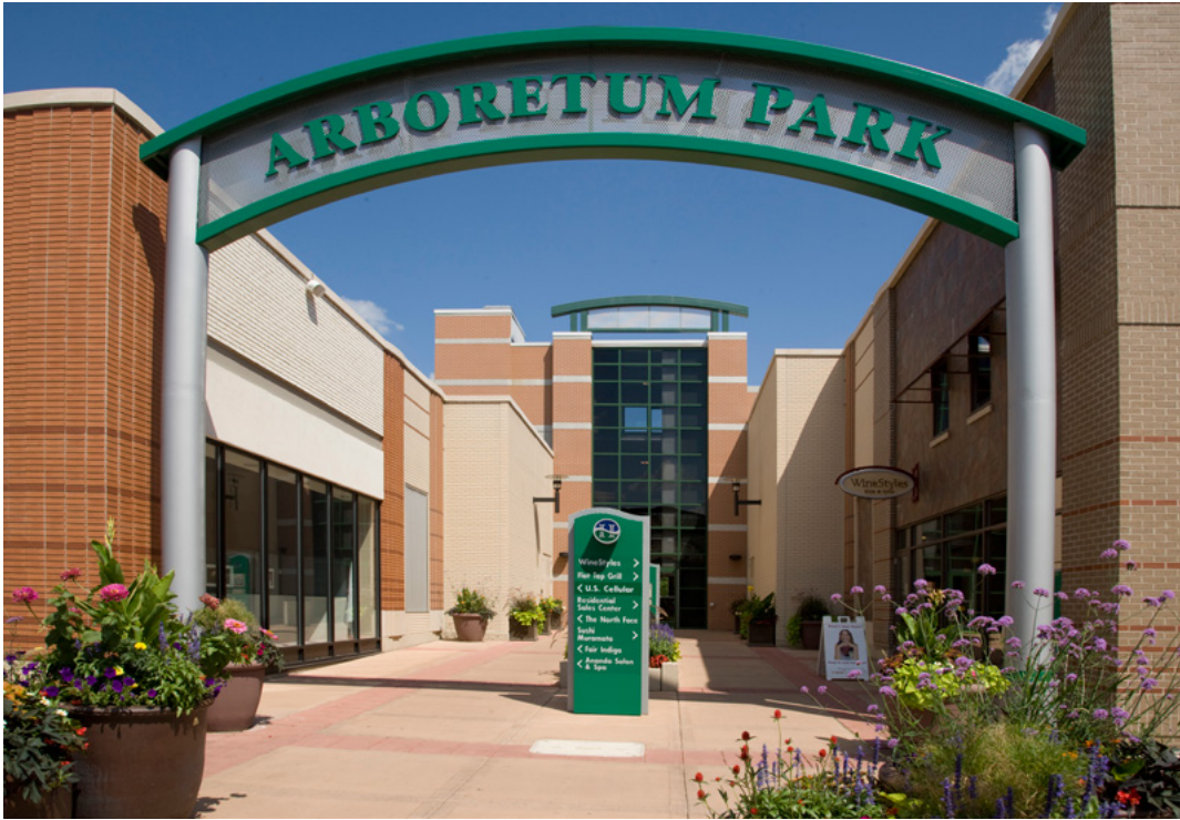
Arboretum Park Garage Entry Sign
