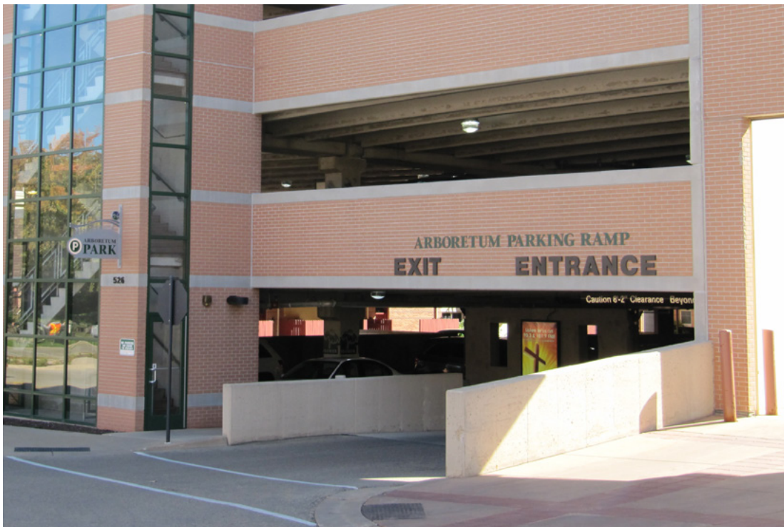
Arboretum Park Garage Entry Wall Sign
