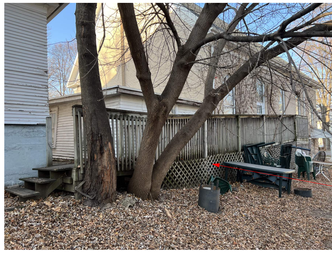
PHOTO 8: EXISTING ACCESSIBLE RAMP TO CHURCH
