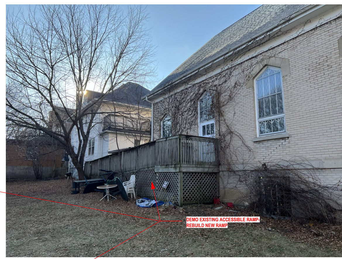
PHOTO 7: EXISTING ACCESSIBLE RAMP TO CHURCH
