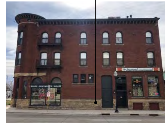
524 E. WILSON ST. FLAT ROOF, MASONRY, BASE WAINSCOT, WINDOW PROPORTIONS, RELATIVE SCALE
