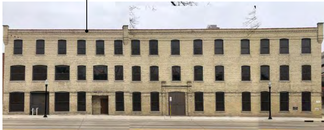
602 RAILROAD ST. FLAT ROOF, MASONRY, WINDOW PROPORTIONS, CORNICE EXPRESSION, RELATIVE SCALE
