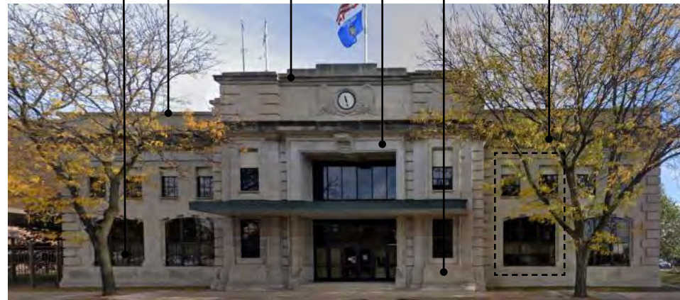
631 RAILROAD ST. FLAT ROOF, MASONRY, DOUBLE-HEIGHT ENTRY EXPRESSION, BASE WAINSCOT, CORNICE EXPRESSION, WINDOW GROUPINGS, RELATIVE SCALE
